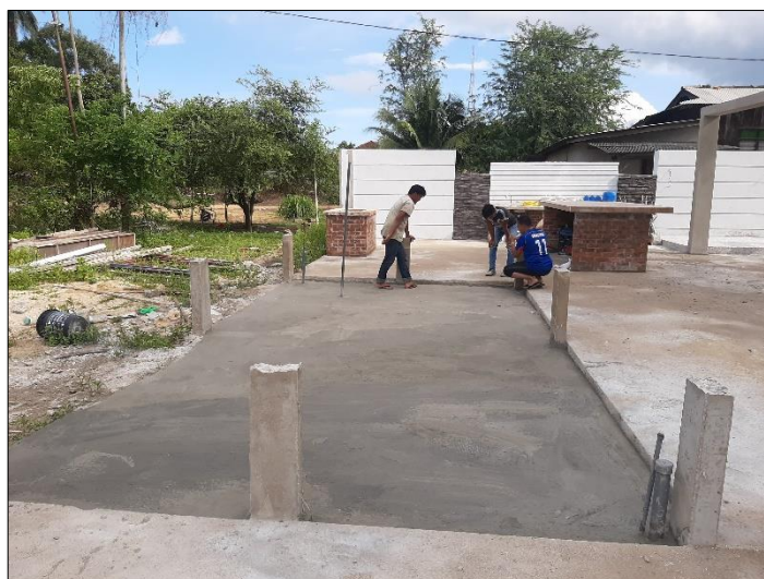
Figure 3.17: Applying waterproof to swimming pool slab
