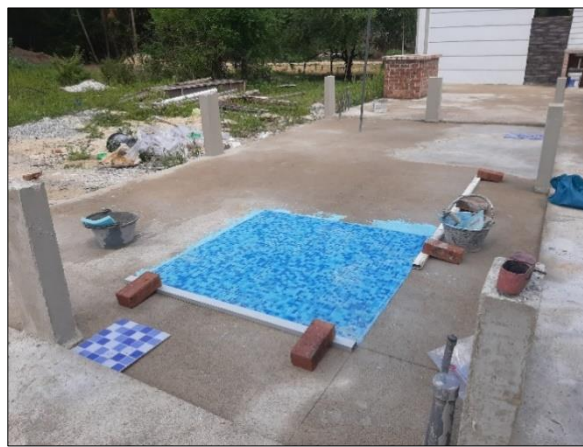
Figure 3.22: set the tile layout for the first quadrant
