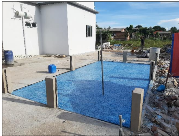
Figure 3.25: mosaic tiles installation complete
