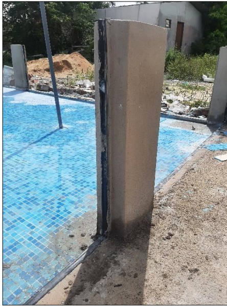
Figure 3.20: plastering work for column completed
