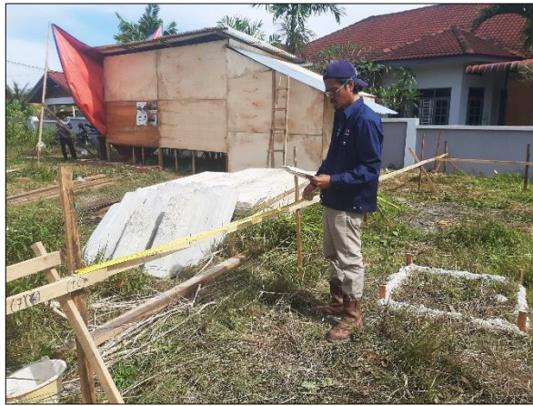
Figure 3.5: Inspection by Site Supervisor for setting out work
