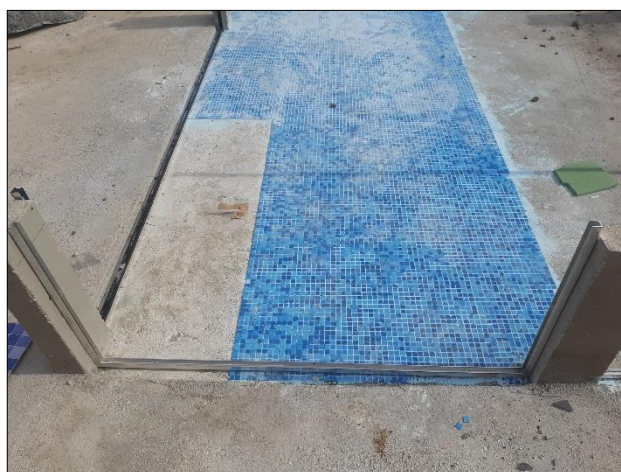
Figure 3.19: Installation of U-shaped aluminium channel
