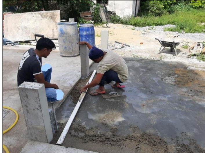
Figure 3.18: Rendering work on the swimming pool floor
