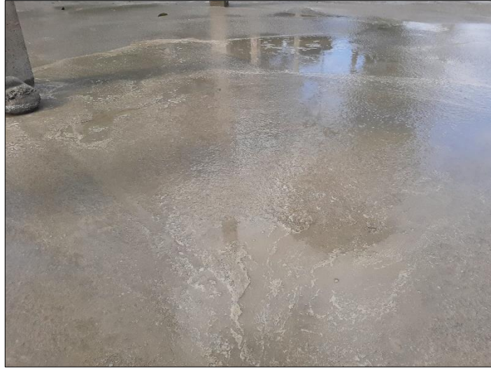
Figure 3.13: screeding work on concrete of swimming pool slab done
