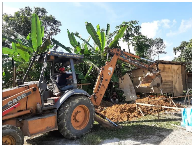
Figure 3.6: Excavation work was done using backhoe
