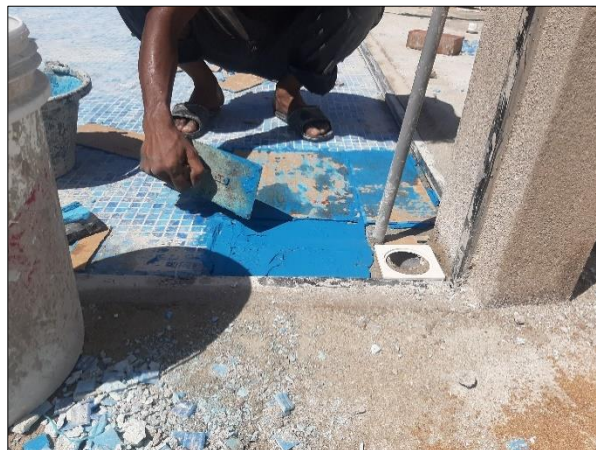
Figure 3.23: installation of a mosaic tile sheet on the adhesive layer
