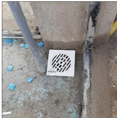
Figure 3.12: Hole outlet installed with floor trap
