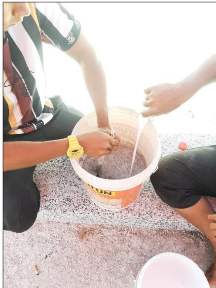
Figure 3.16: Mixing the Component A and B
