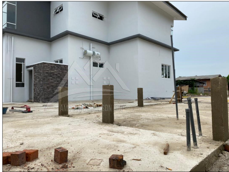
Figure 3.14: Completed process of concrete work
