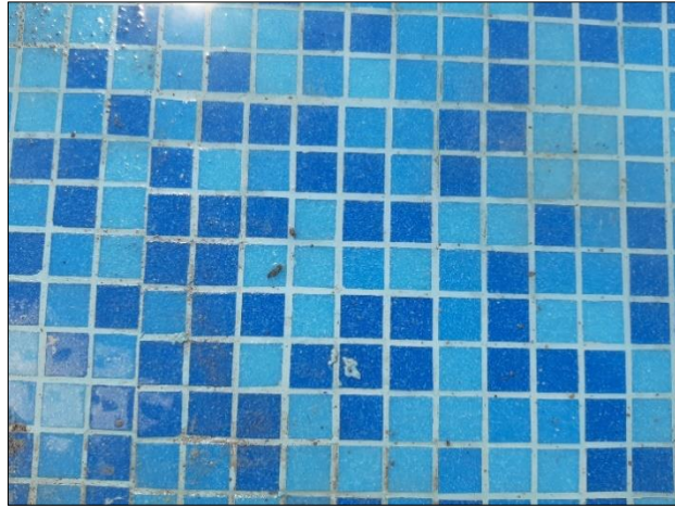
Figure 3.24: Grouting on the mosaic tile completed
