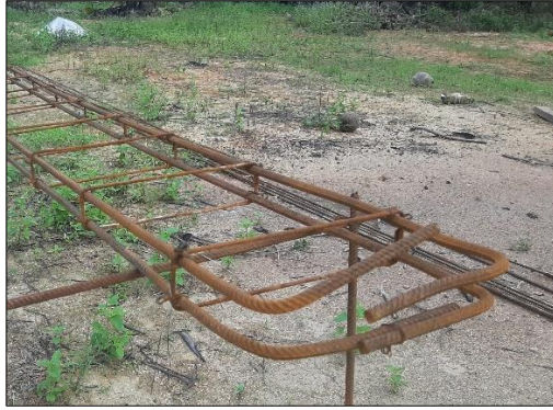
Figure 3.8: Casting of the column reinforcement
