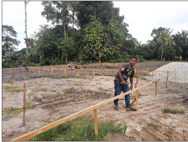
Figure 3.4: workers installed profile boards
