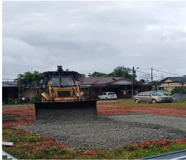
Photo 3.3.3 Cover the excavated area with pebbles Port Klang, Selangor
