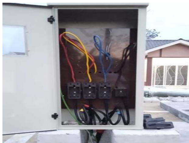
Photo 3.3.10 Installing the TNB metre box
