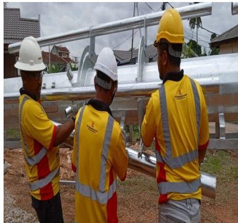
Photo 3.3.15 Installing the boom the boom slot
