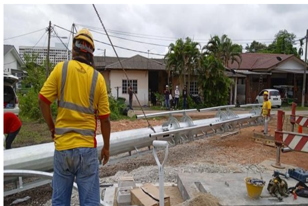
Photo 3.3.17 Tie the sling belt to pole
