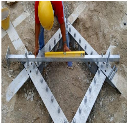
Photo 3.3.8 check the level with leveller
