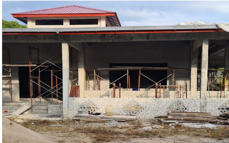
Photo 2.4.3 Construction of Mussola at SMK Desa Cempaka
