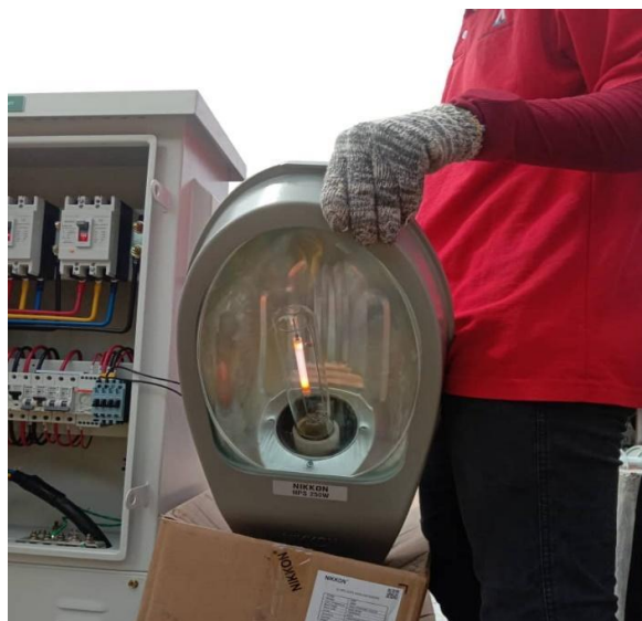
Photo 3.3.13 Testing Street light
