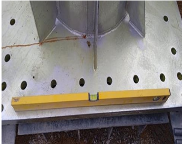
Photo 3.3.20 Check the level of each side
