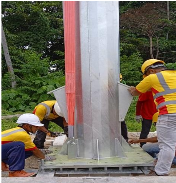
Photo 3.3.19 Help the crane to put pole in its slot
