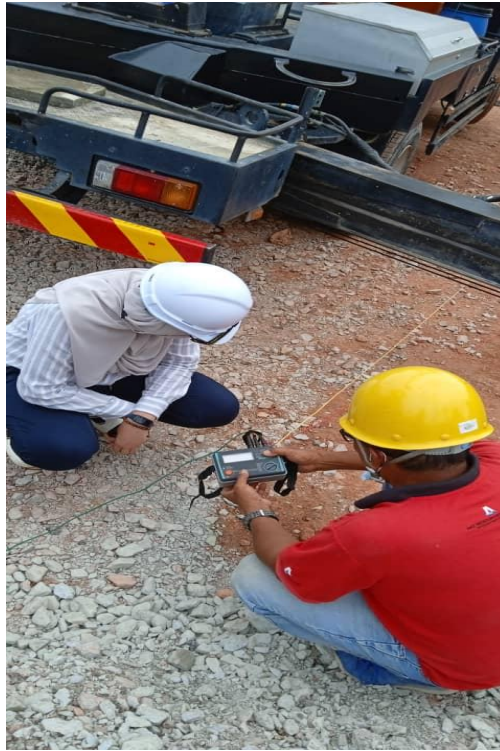
Photo 3.3.25 Check the grounding electricity
