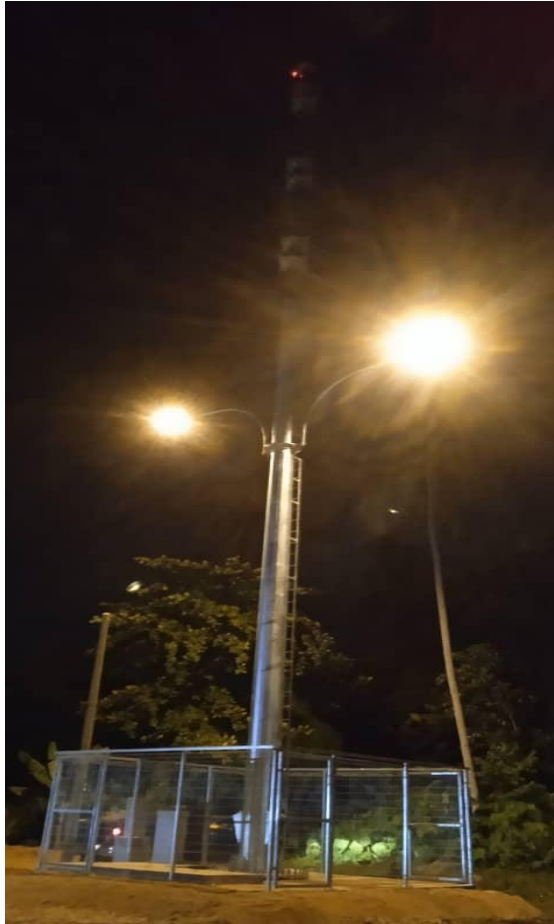
Photo 3.3.28 Completed Telecommunication Pole
