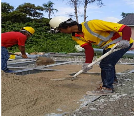
Photo 3.3.6 Cover the surface with sands
