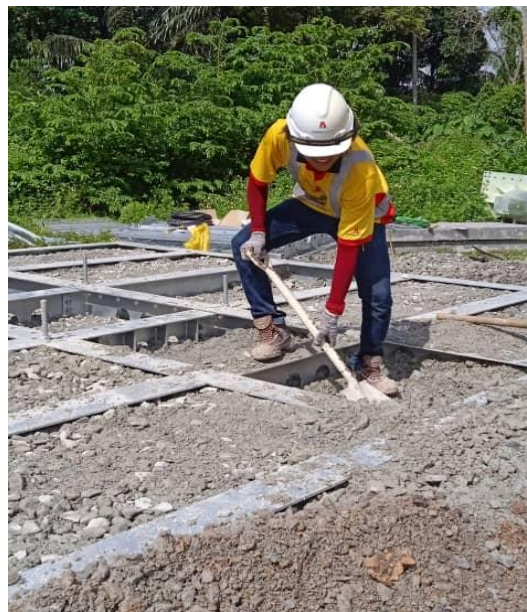
Photo 3.3.5 Filling the base with pebbles
