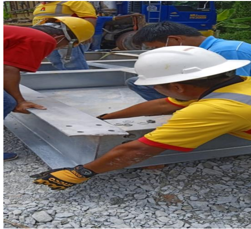
Photo 3.3.4 Installing the TLP base
