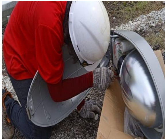
Photo 3.3.12 Wiring the street light
