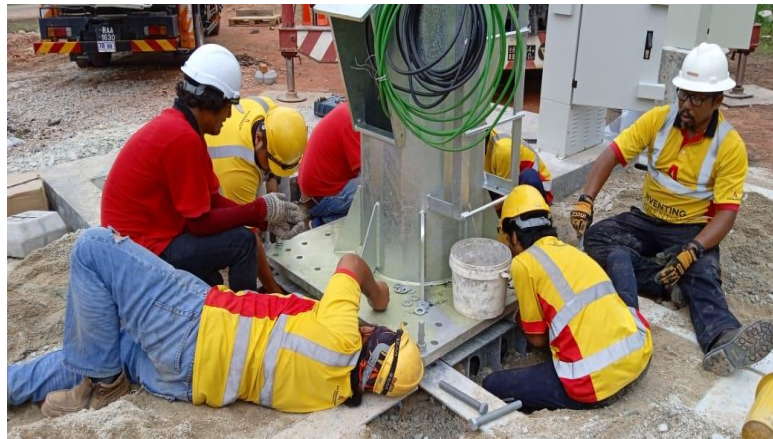
Photo 3.3.21 Screwed the nut from base to bottom pole
