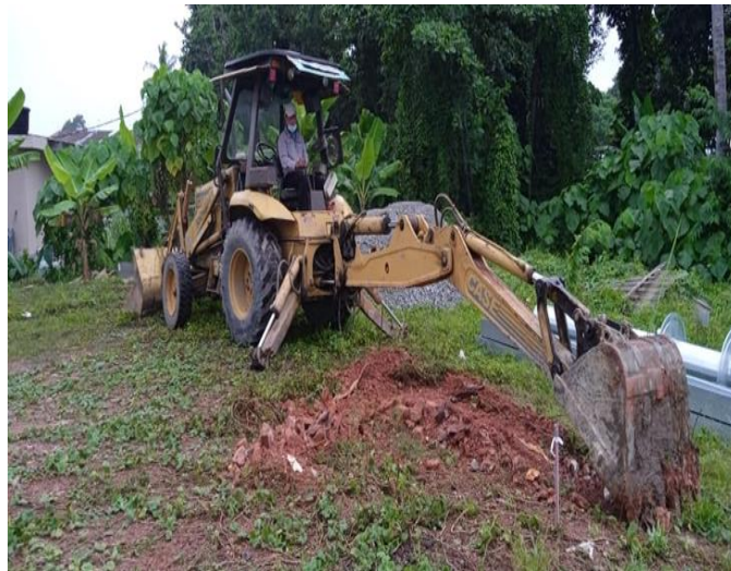
Photo 3.3.2 Excavate the soil using backhoe, Port Klang, Selangor
