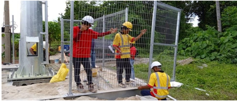
Photo 3.3.26 Installing the fences
