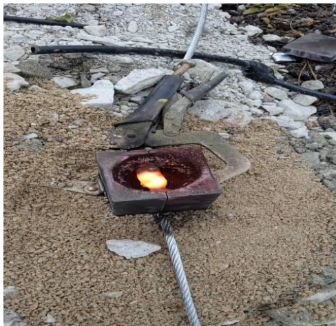
Photo 3.3.24 Seal copper grounding wire to grounding rod using Grounding Box set
