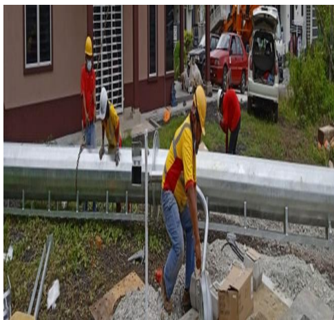
Photo 3.3.16 Installed Street light to pole
