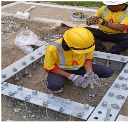
Photo 3.3.7 Installing nuts in middle base for TLP
