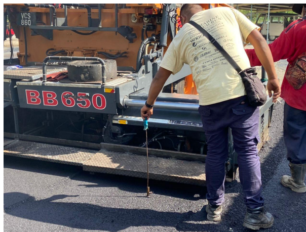
Figure 3.2.6 Measure the thickness of premix before compact
