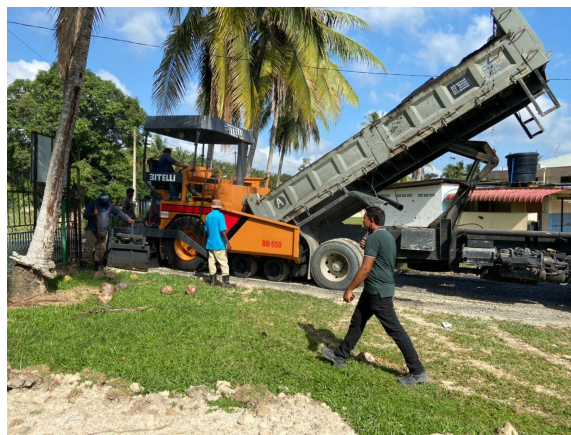
Figure 3.2.4 Workers are pouring premix into the paver from the quarry
