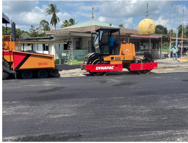
Figure 3.2.7 The worker is compacting the premix
