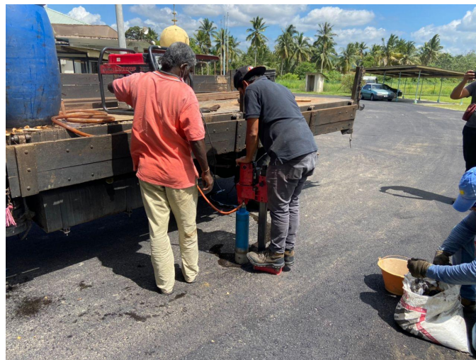
Figure 3.3.1 The workers are doing coring test
