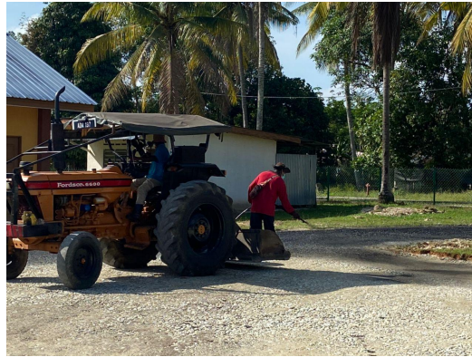
Figure 3.2.3 Worker is watering tack coat on crusher-run
