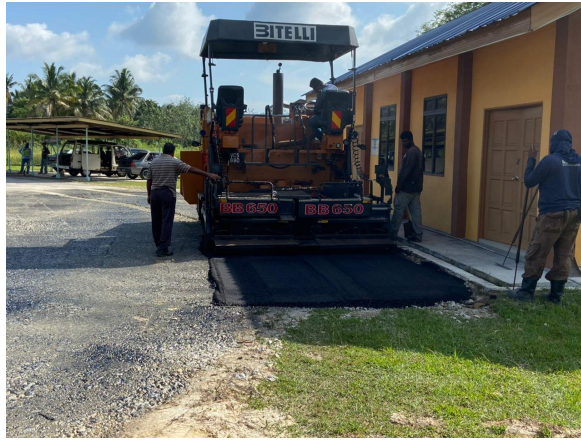
Figure 3.2.5 Workers is pouring premix using paver
