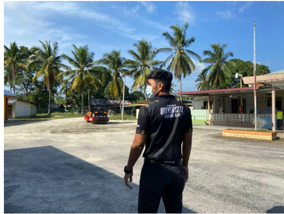
Figure 3.2.1 Checking the original sites to make premix works
