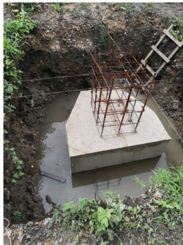
Figure 3.16 & 3.17: Pile caps
