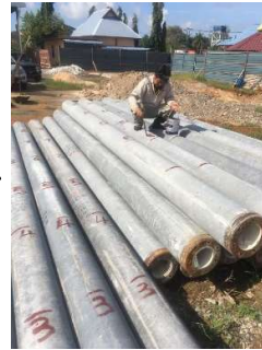
Marking the spun piles
