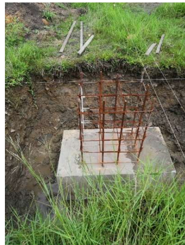
Figure 3.16 & 3.17: Pile caps
