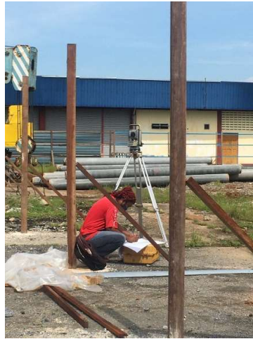
Figure 3.4: Setting Out process
