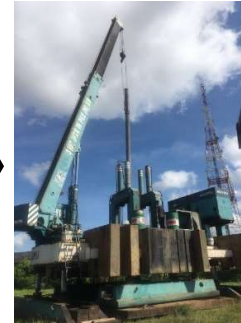
Driving process (Lifting the spun piles)
