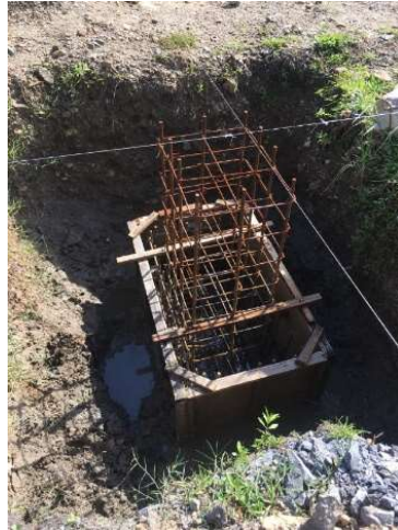
Figure 3.15: Construct formwork for pile cap
