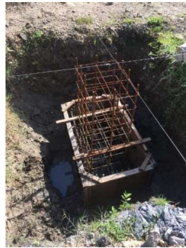
Formwork for pile cap
