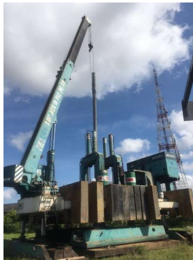
Figure 3.9: Jack-in pile machine (Lifting process)
