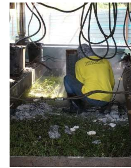
Pile jointing and cut off the excess pile head
