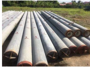
Delivery of spun piles
