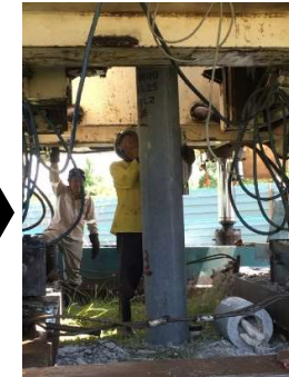
Get correct vertical level of spun piles
