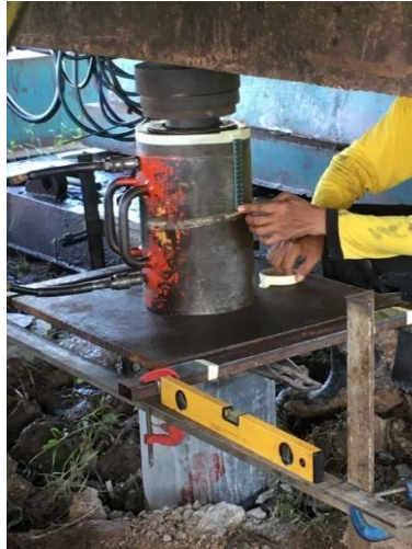
Figure 3.13: Attachment scale at test pile
