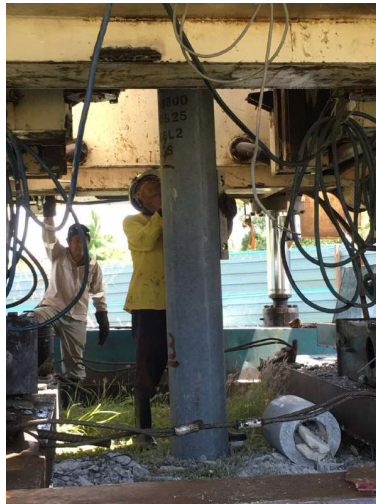
Figure 3.10: Used spirit level to get correct vertical level
