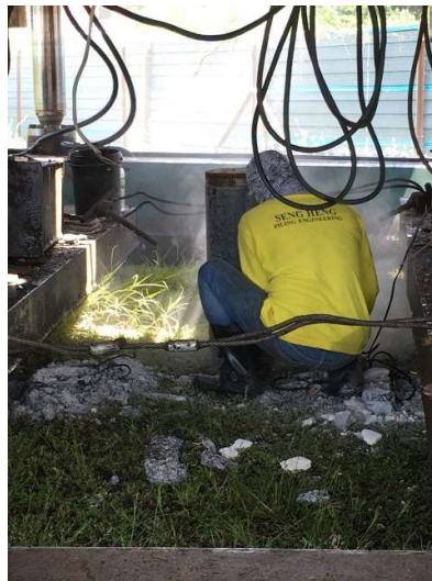
Figure 3.11: Cut off the excess pile head
