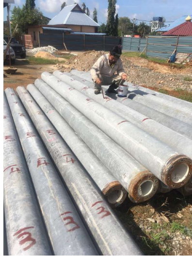
Figure 3.8: Marking the spun piles
