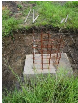
Construct pile cap
