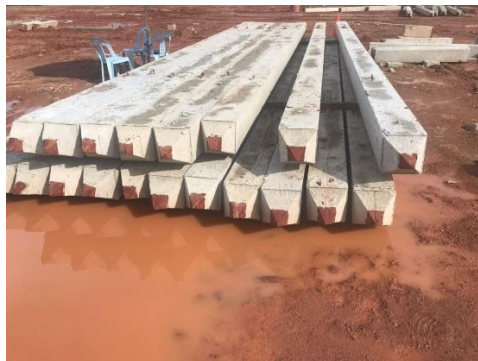
Figure 11: 250x250mm RC pile (starter)
