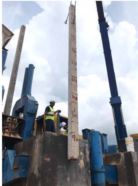
Figure 15: Marked pile
