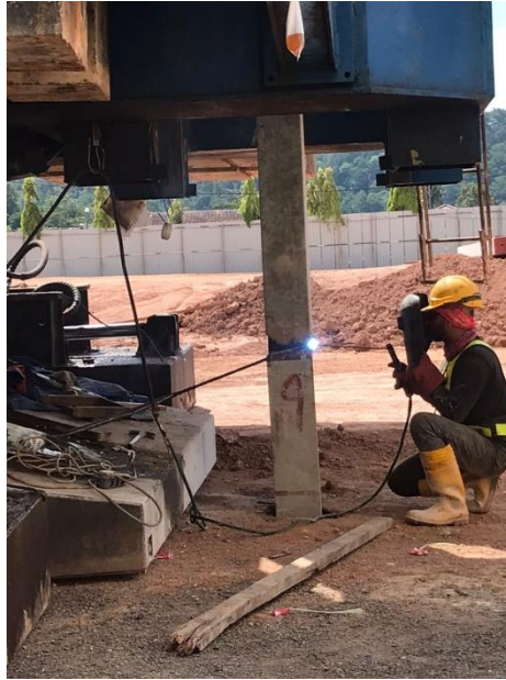
Figure 20: butt welding
