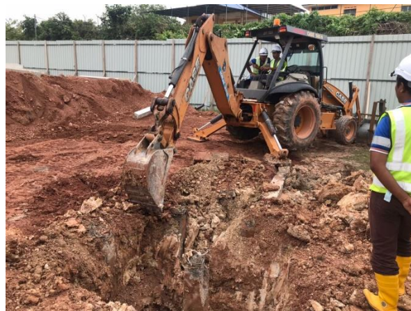
Figure 26: preparation for PDA test
