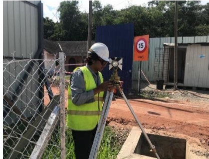
Figure 13: Setting out piling point
