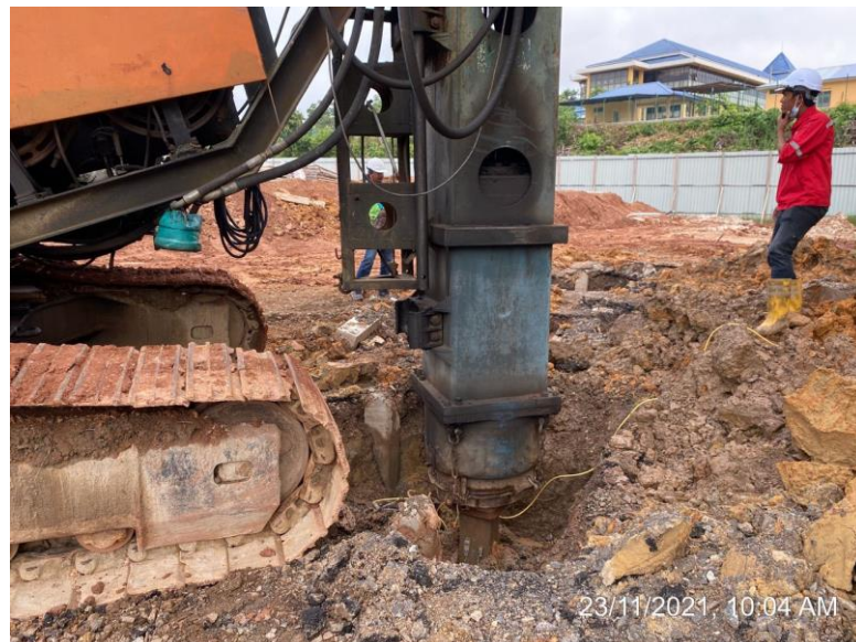
Figure 31: Setting up of hammer
