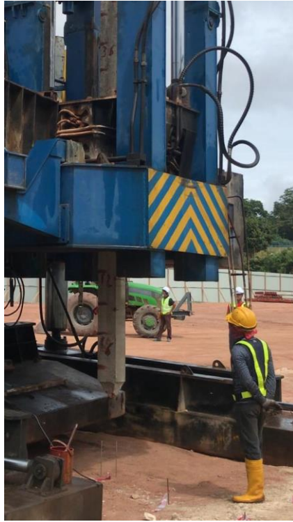
Figure 18: Setting out piling on the piling point
