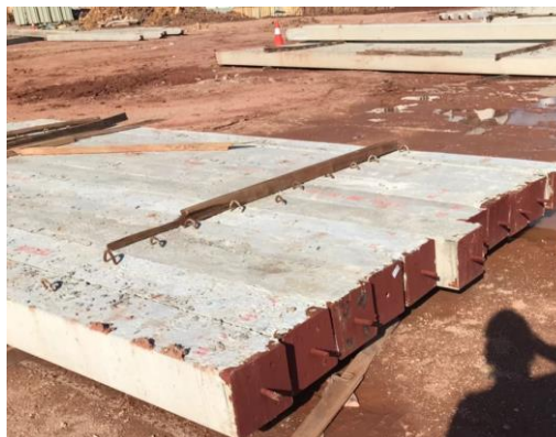
Figure 12: 250x250mm RC pile (extension)
