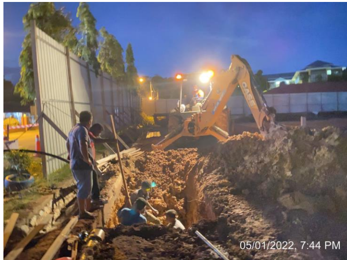
Figure 34: Fixing pipe work
