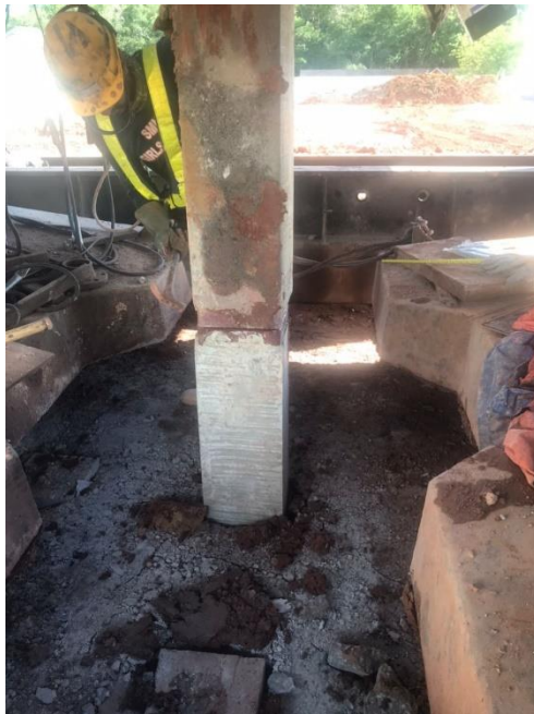
Figure 19: installation of extension pile
