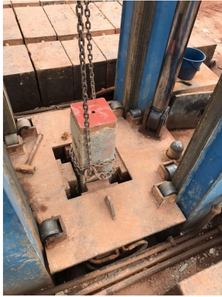
Figure 16: Piling in griped position
