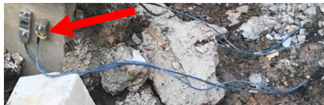
Figure 28: Strain Transducers and Accelerometers
