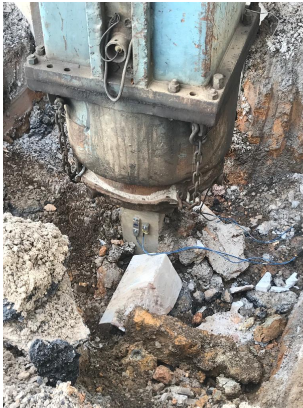
Figure 30: Installation of Strain Transducers and Accelerometers
