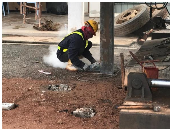
Figure 23: Cutting the balanced piling
