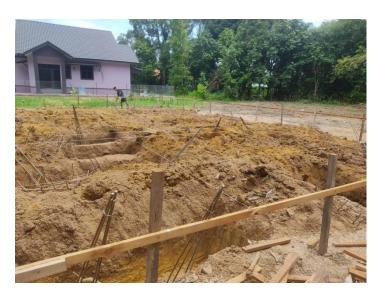
Figure 3.6 Setting Out for Column
