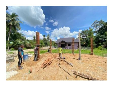
Figure 3.10 Completed Column
