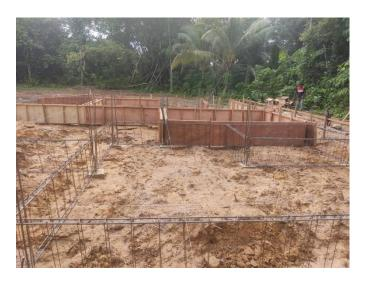
Figure 3.3 Ground Beam Formwork
