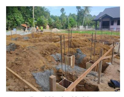
Figure 3.7 Reinforced for Column
