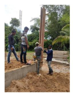
Figure 3.8 Formwork for Column
