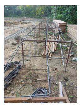
Figure 3.1 Arranging the Rods
