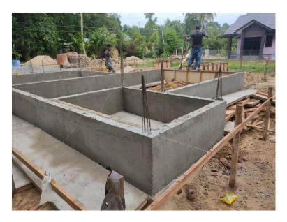
Figure 3.5 Complete Ground Beam
