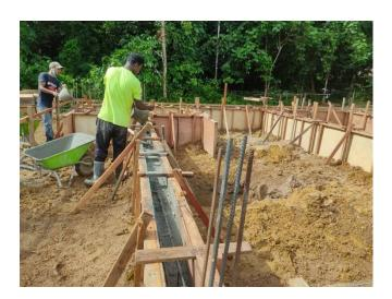
Figure 3.4 Pouring the Concrete
