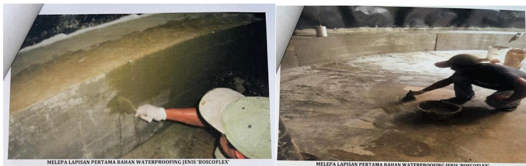
Figure 3.4.3 First layer of waterproofing works
