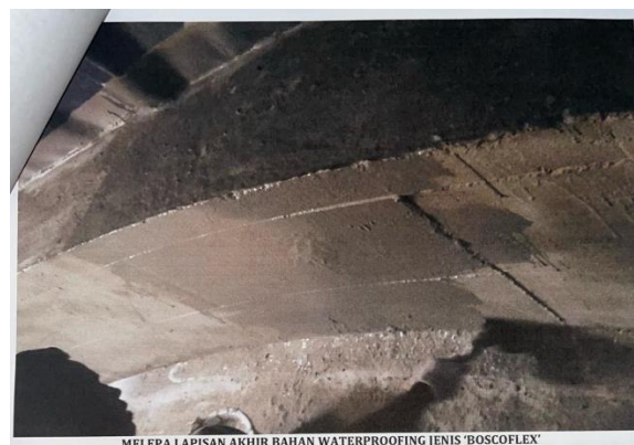
Figure 3.4.7 After 3-6 hours, apply the last layer of Boscoflex waterproofing
