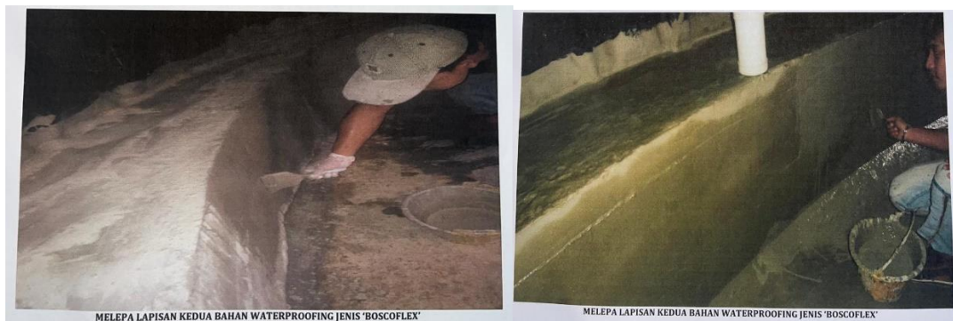
Figure 3.4.4 Second layer of waterproofing works
