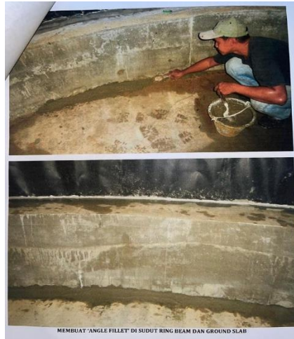
Figure 3.4.2 Angle fillet works
