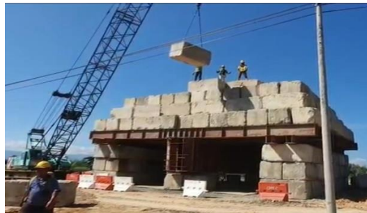
Figure 3.3.6 Load the kentledge blocks
