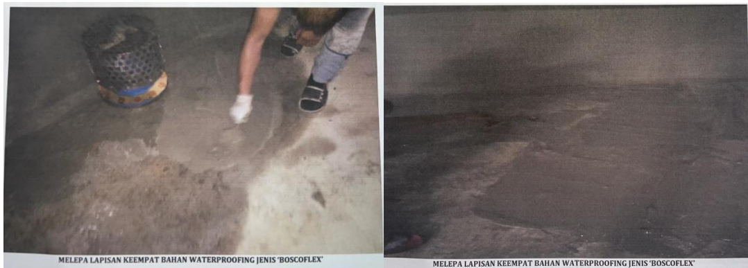
Figure 3.4.6 Fourth layer of waterproofing works
