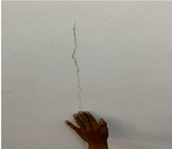
Figure 6 : scrap the crack
