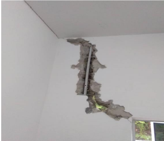
Figure 4 : Wall has been hacked by demolition hammer
