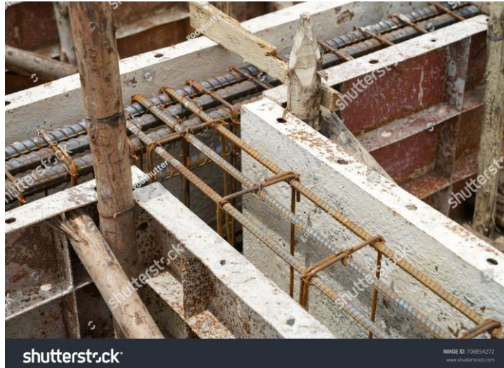
Figure 3.8: Example of reinforcement bar in roof beam
