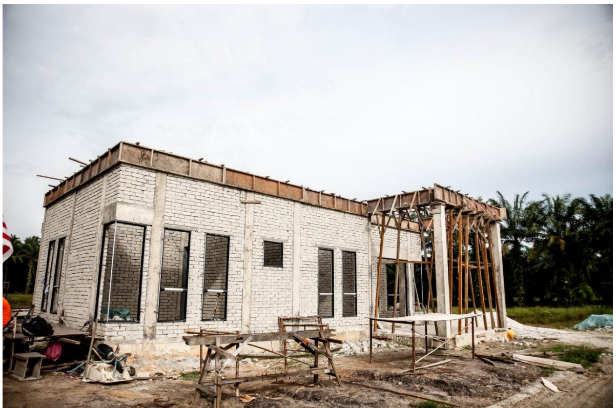
Figure 3.5: Process Installation of Roof Beam at Site Chenderong Balai.
