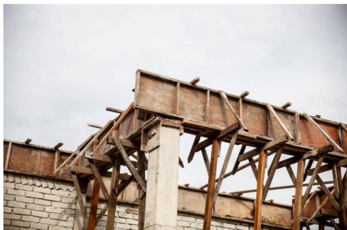
Figure 3.7: Formwork of Roof Beam
