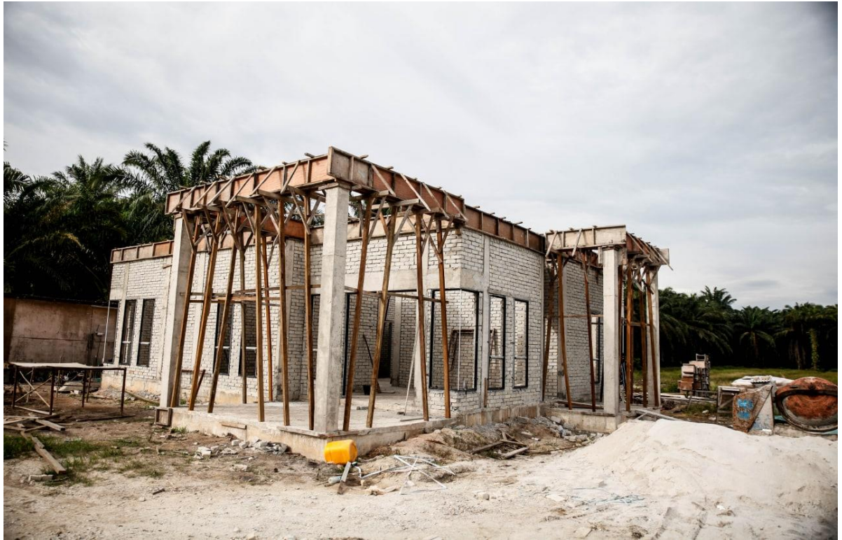
Figure 3.4 : Process Installation of Roof Beam at Site Chenderong Balai.
