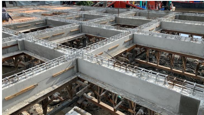
Figure 3.10 : Example of concreting work of roof beam.
