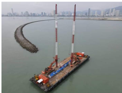
Figure 3.1.1 PVD work project Tanjung Tokong STP 2
