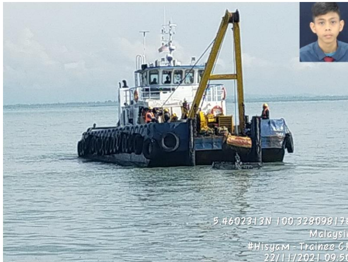
Figure 3.2.6 Change Anchor Barge to New Position with Tug Boat
