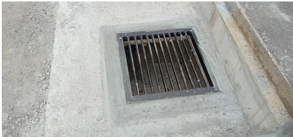
Figure 1.26: Drain grating to close holes in concrete
