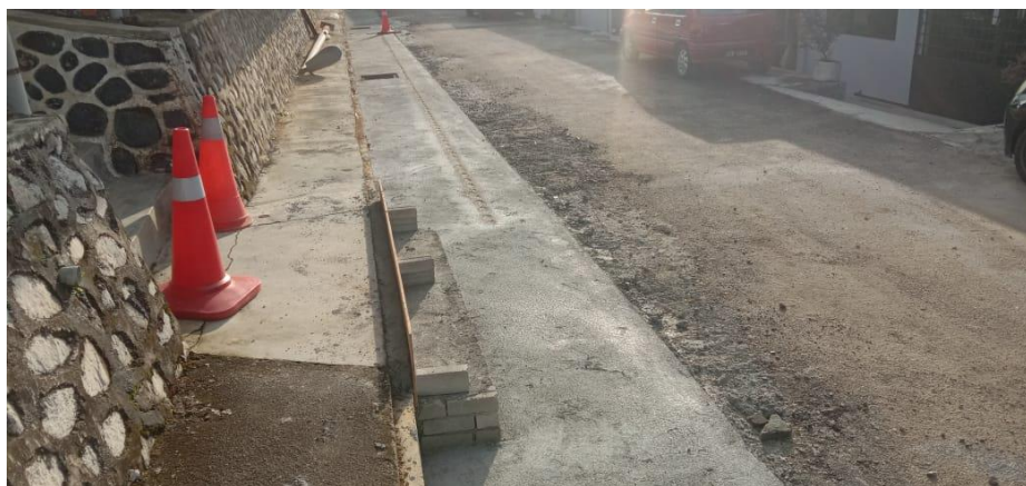
Figure 1.27: Areas that have been concreted
