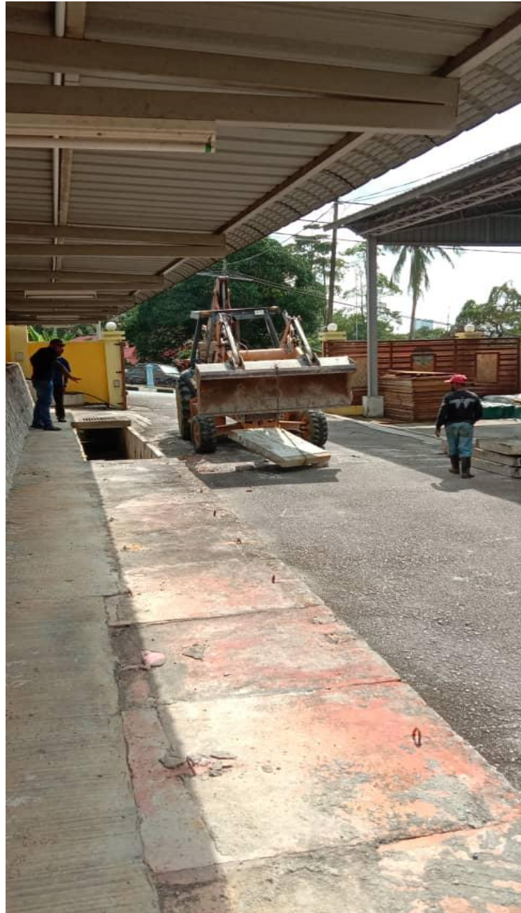
Figure 1.15: Lifting concrete drainage cover
