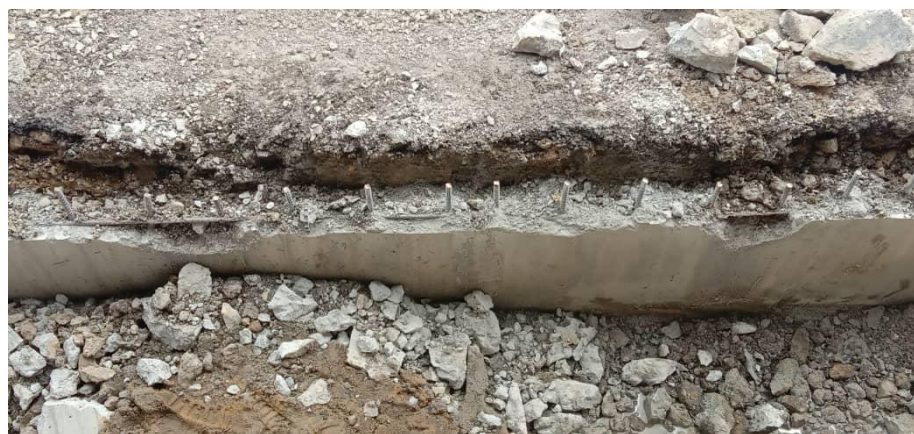
Figure 1.22: Steel reinforcement after cutting
