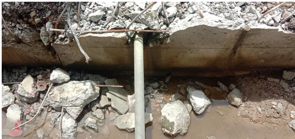
Figure 1.19: Results after the culvert box is broken using a backhoe
