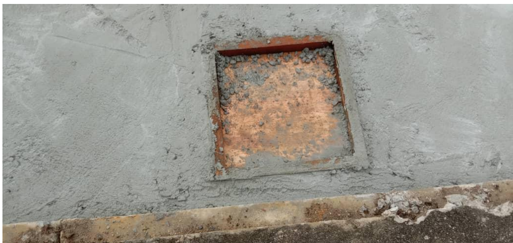
Figure 1.24: Formwork for grating installation
