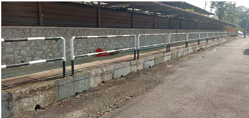
Figure 1.13: Picture before the iron railing was opened.
