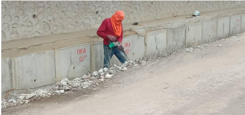
Figure 1.20: Workers holding a hammer machine breaker
