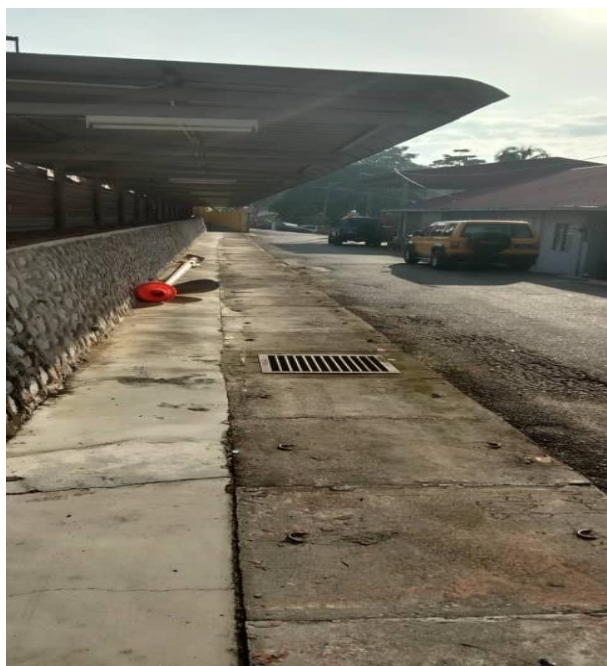
Figure 1.14: Picture after the iron railing was opened
