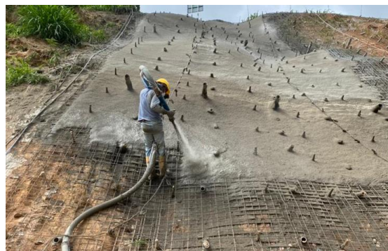
Figure 4.3 Technique of spraying guniting
