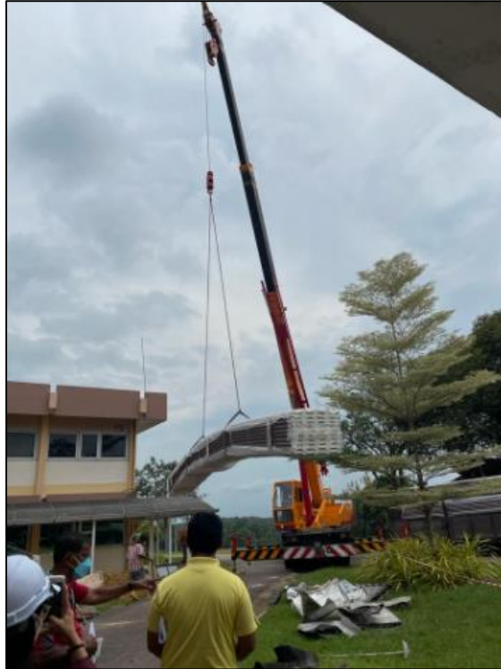
Figure 3.18: Metal deck roofing sheets are lifted using a crane
