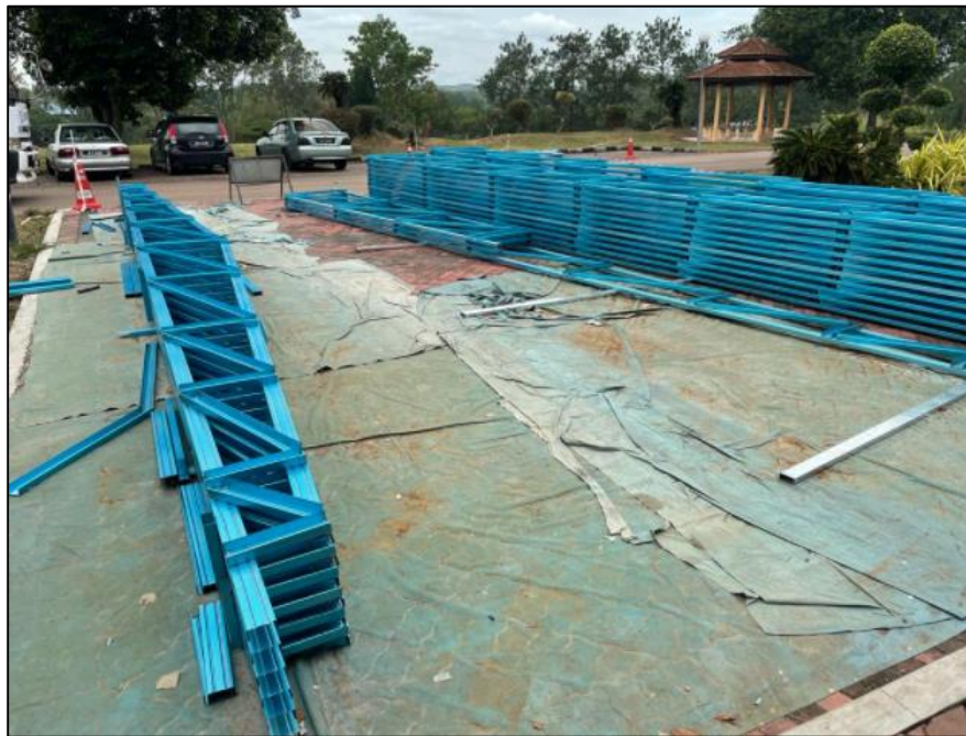
Figure 3.17: The roof trusses are stacked before being covered with canvas
