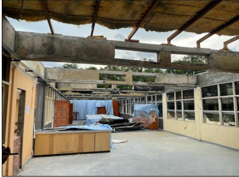
Figure 3.15: Meeting room view after dismantling the roof insulation foam
