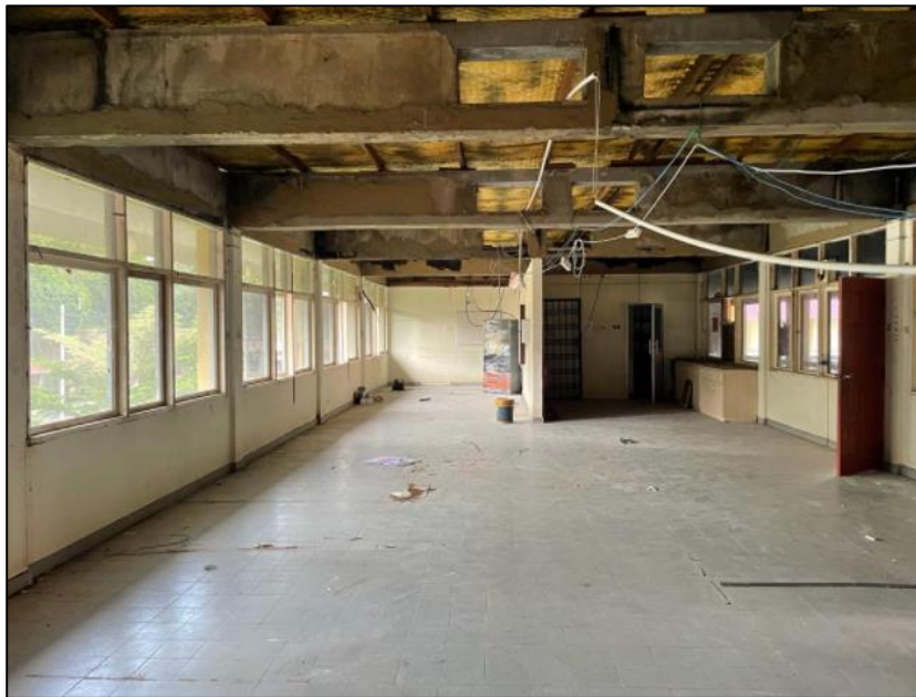
Figure 3.14: Staff office view after dismantling the ceiling structure
