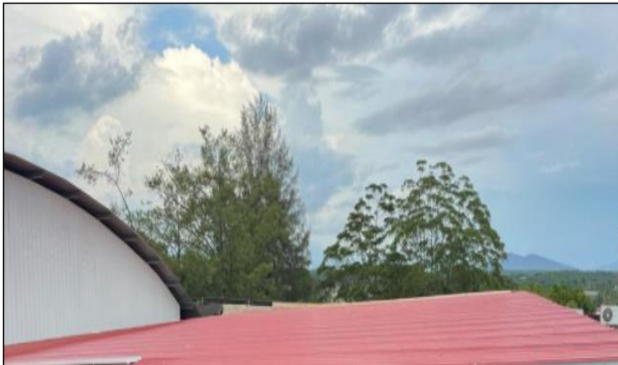
Figure 3.11: Red metal deck sheet roofing
