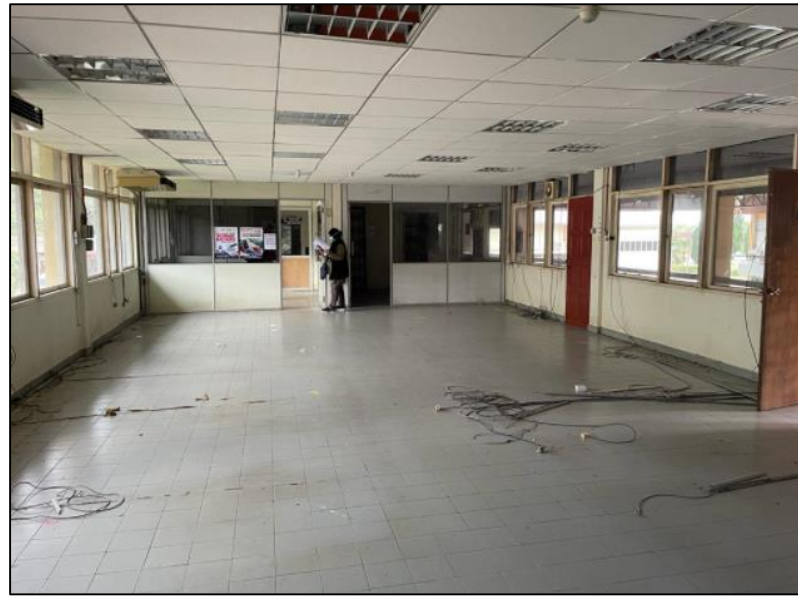
Figure 3.7: Staff office ceiling
