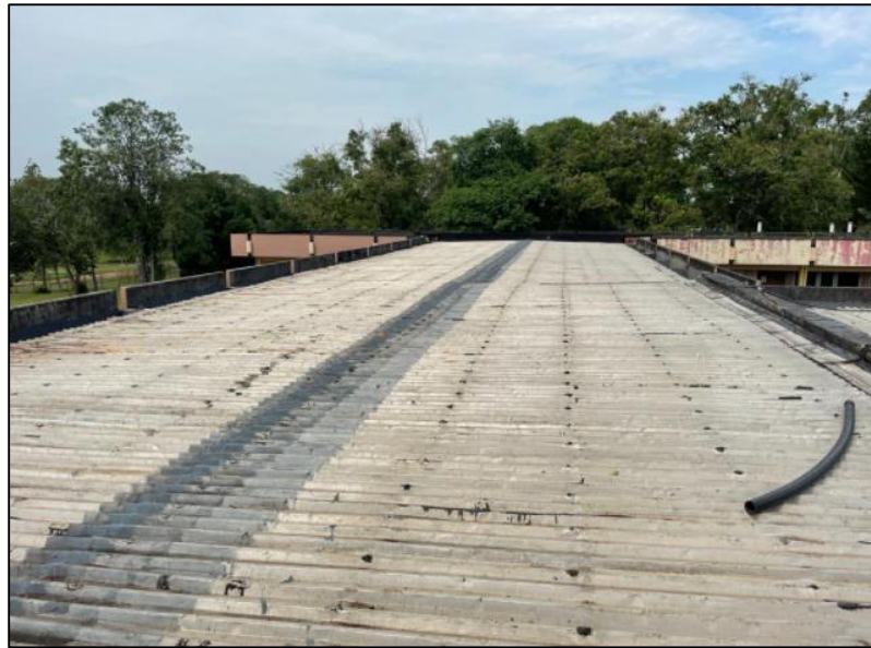
Figure 3.9: MVI administrative block roof
