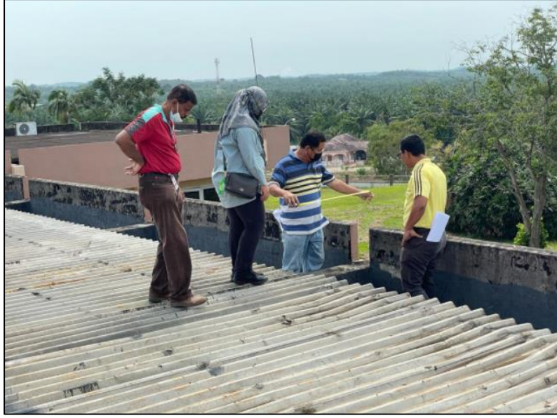
Figure 3.8: Inspection work on the MVI administrative block roof
