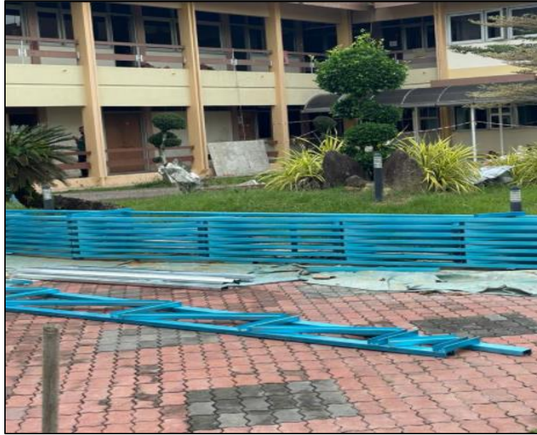
Figure 3.12: Steel roof trusses
