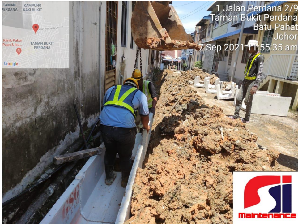
Figure 3.2.2 Installing the drain
