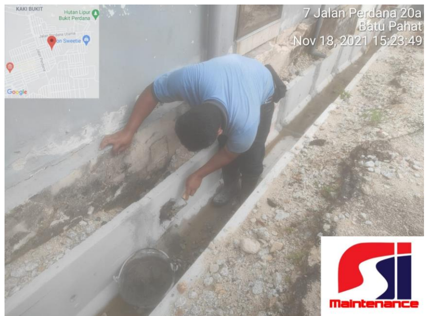
Figure 3.2.3(2) Plaster the gap between drain
