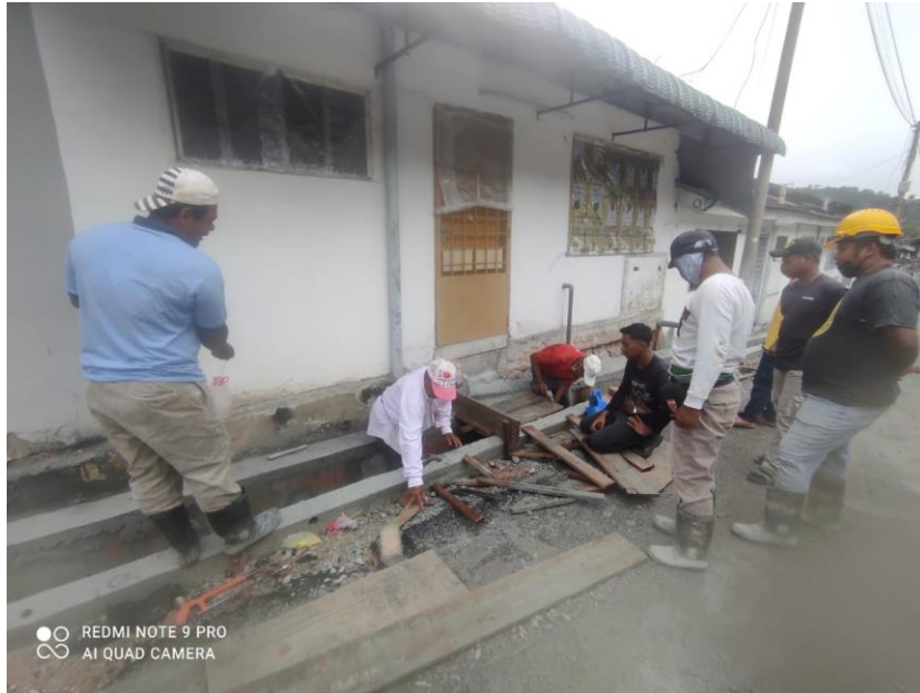
Figure 3.2.4(3) remove the formwork
