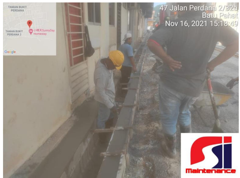
Figure 3.2.4(2) concrete the beam
