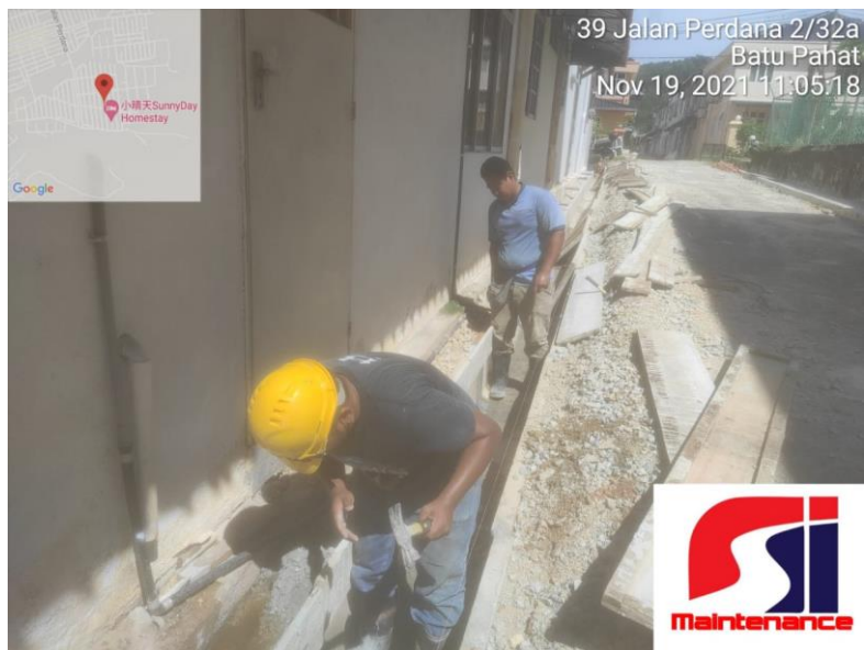
Figure 3.2.4(1) install the formwork
