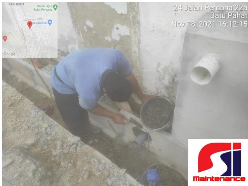
Figure 3.2.3(1) Plaster around the pipe
