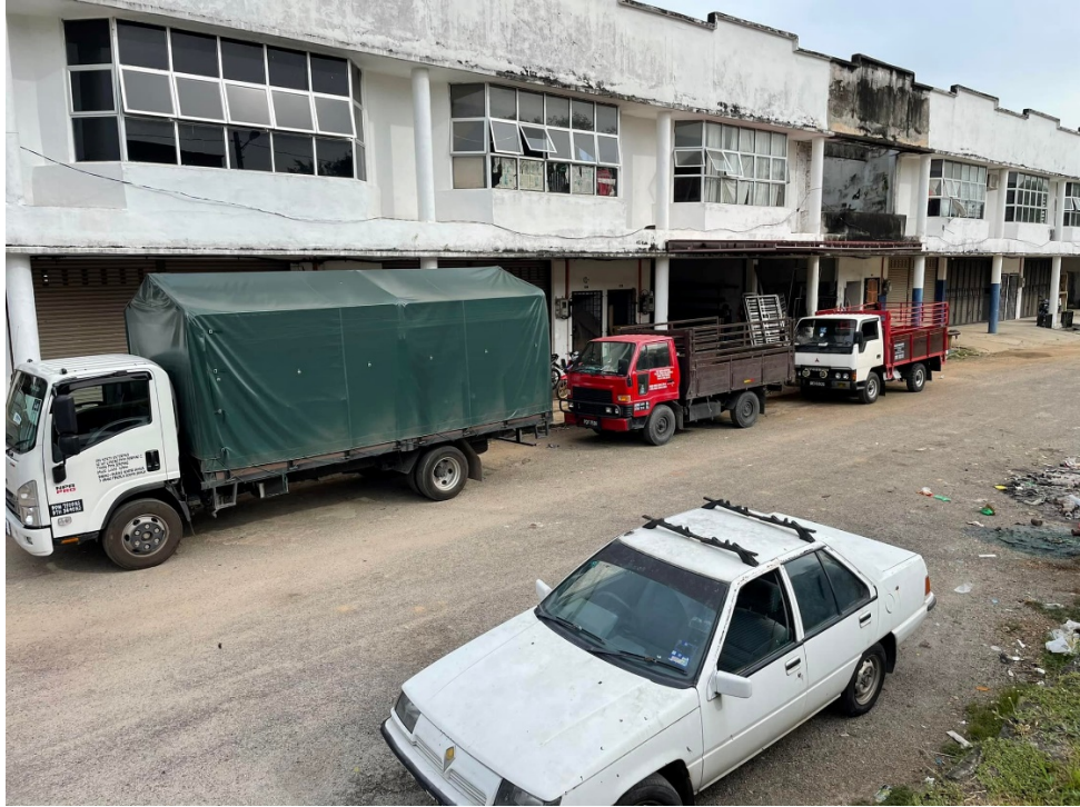
Figure 2.1: Front view of the office and workshop
