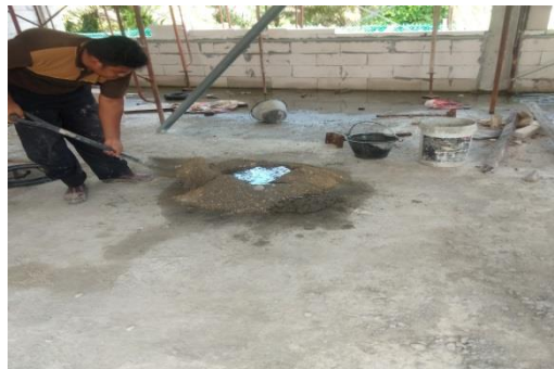
Figure 3.2.2 The mix of cement mortar
