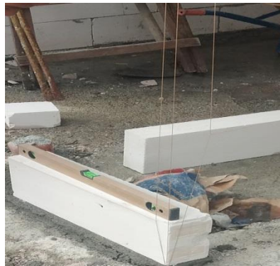
Figure 3.2.3 pin and guide line
