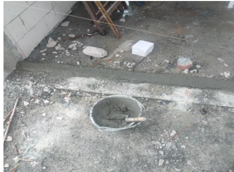
Figure 3.2.4 laid of rough concrete
