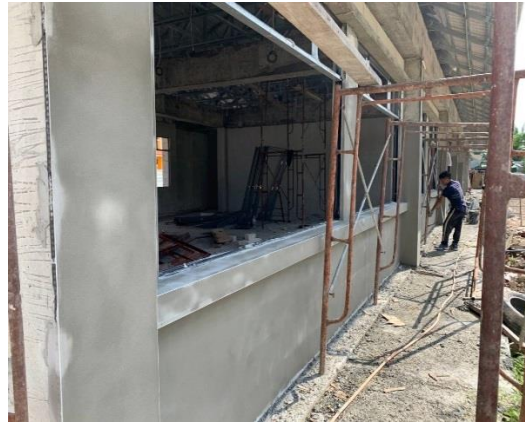
Figure 3.2.9 plastering work( finishes touches)
