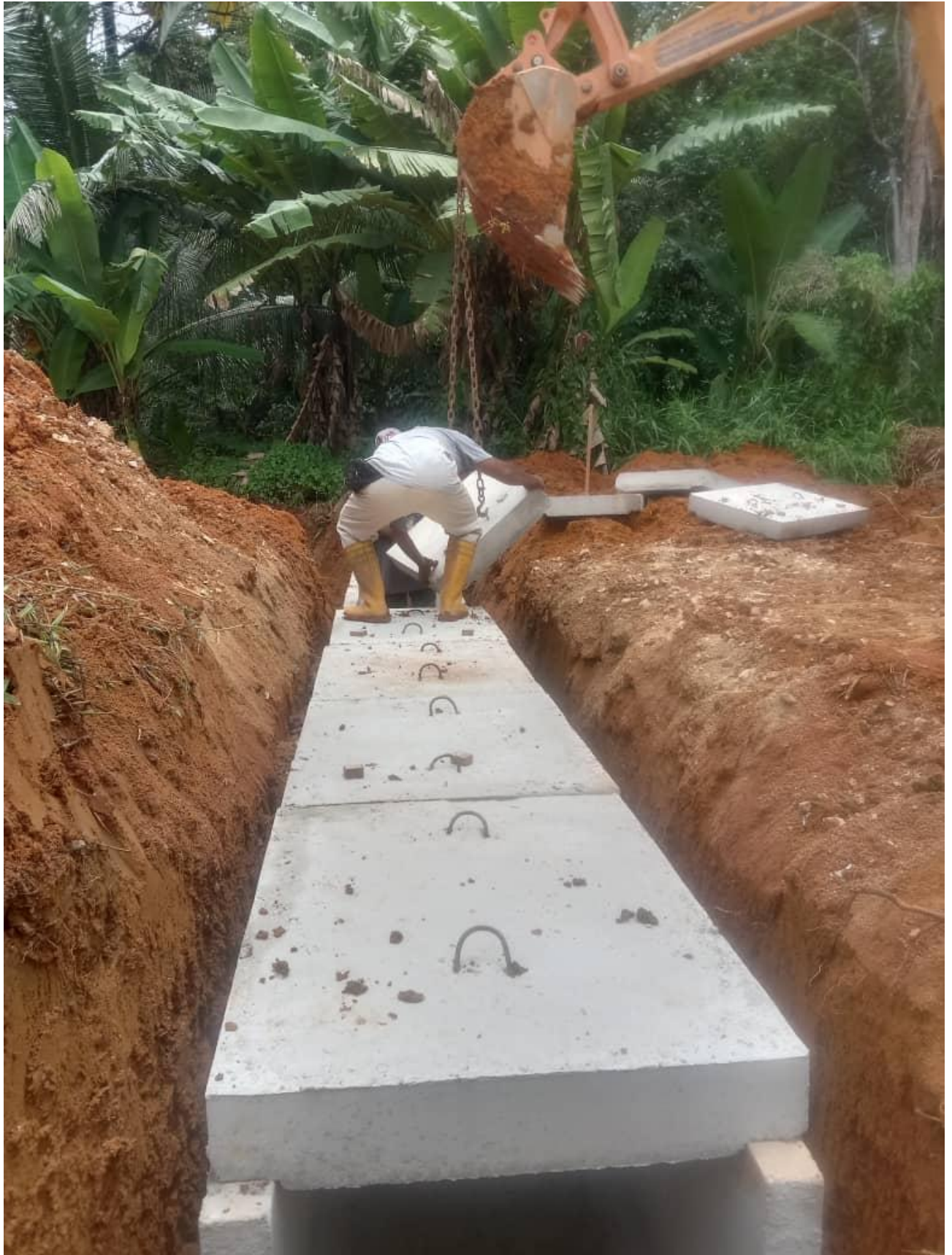
Figure: installing the drainage at chaah
