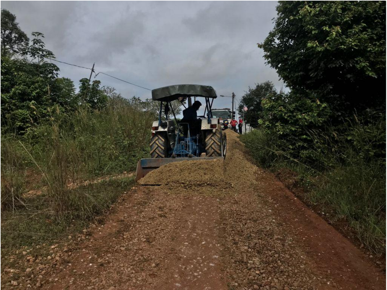
Figure: pouring crusher run over the Bukit Siput main road
