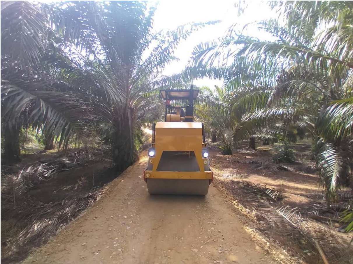
Figure: compacting the Paya Terap road
