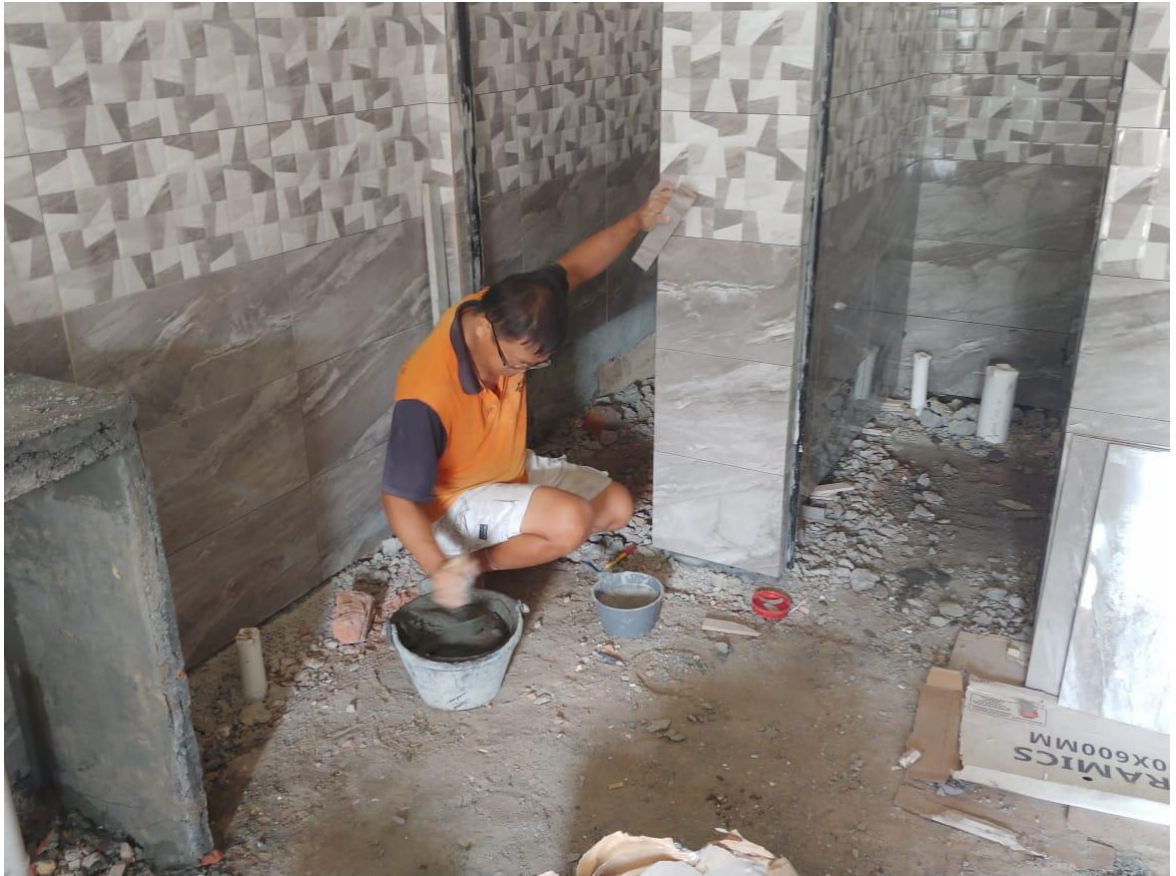
Figure: installing the ceramic tiles on the mensudut pindah school toilet floor
