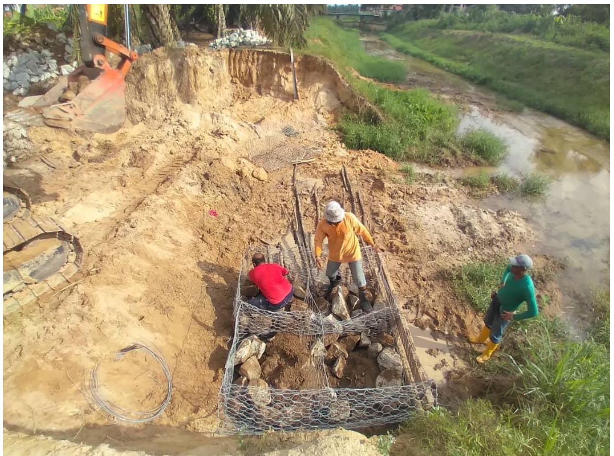
Figure: arranging the rock at Lubuk Bandan river
