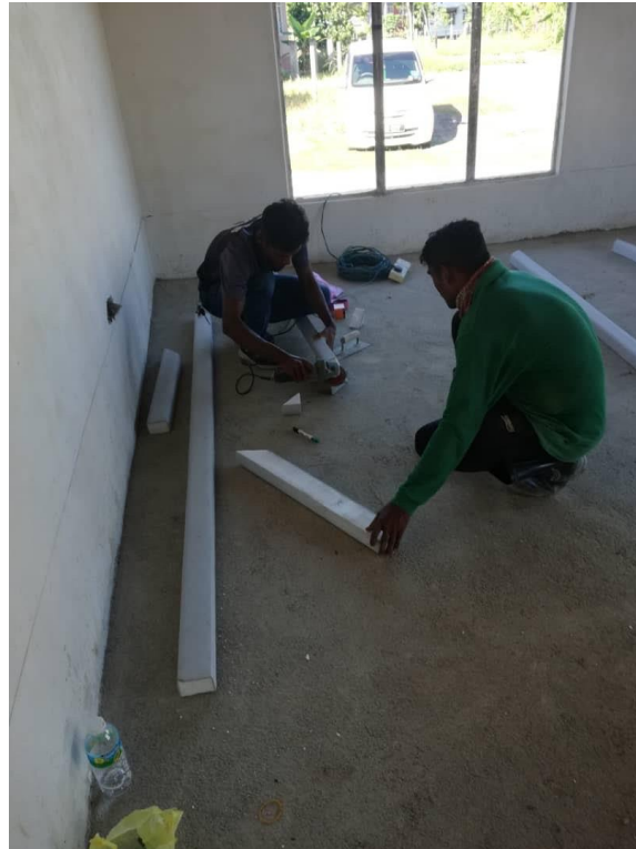
Figure 3.14 Worker cutting the coping
