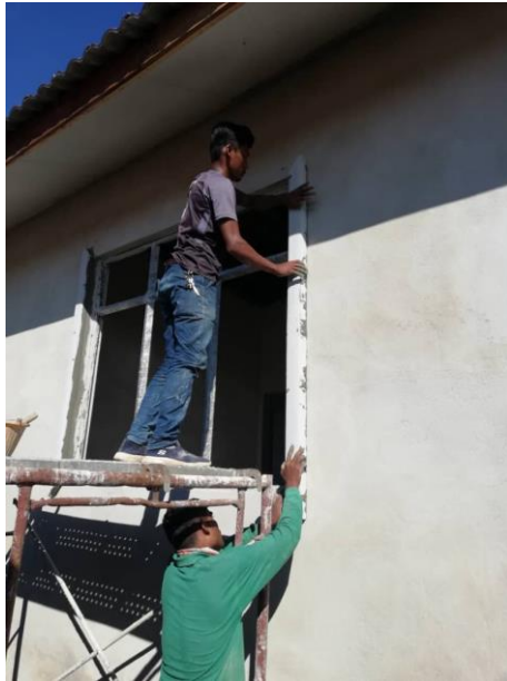
Figure 3.15 Worker place the coping.
