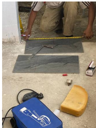
Figure 3.18 Worker cut the tile.
