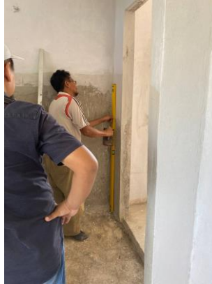
Figure 3.17 Worker check the wall.
