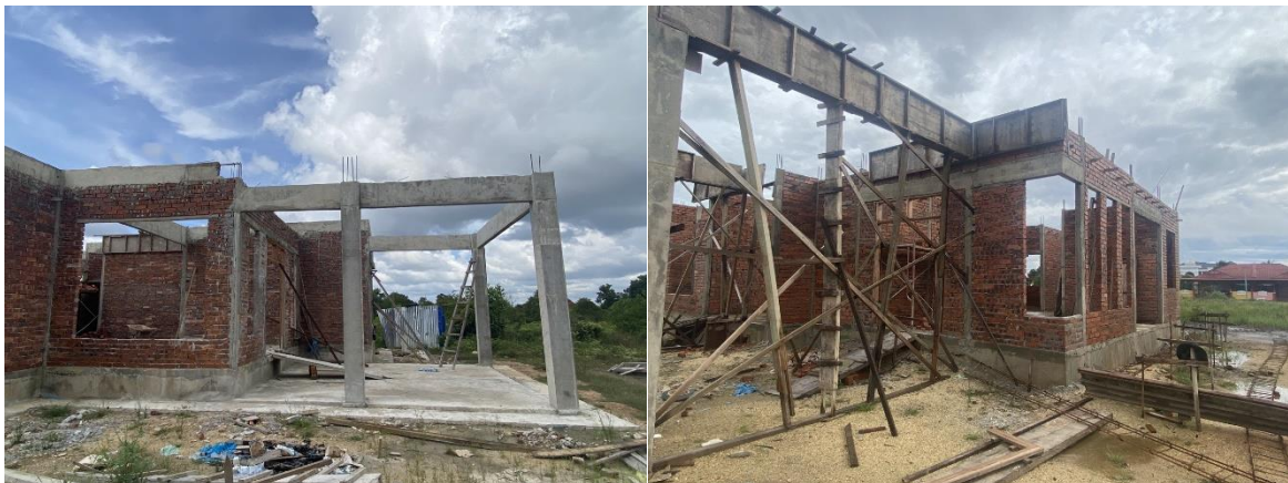
Figure 3. 23 Roof beam inspections at site Kubang Parit.
