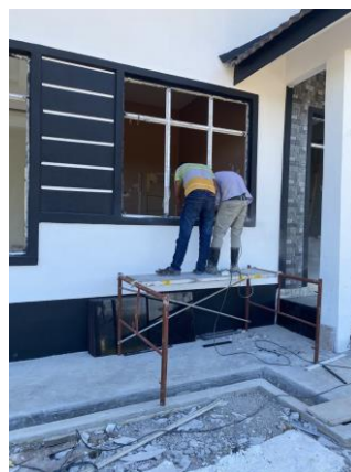
Figure 3.29 Worker fix the coping.
