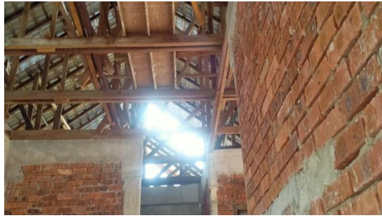
Figure 3.24 Roof construction at site Durian Burung.
