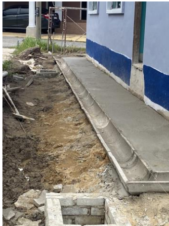
Figure 3.20 Drains at site Atas Tol.
