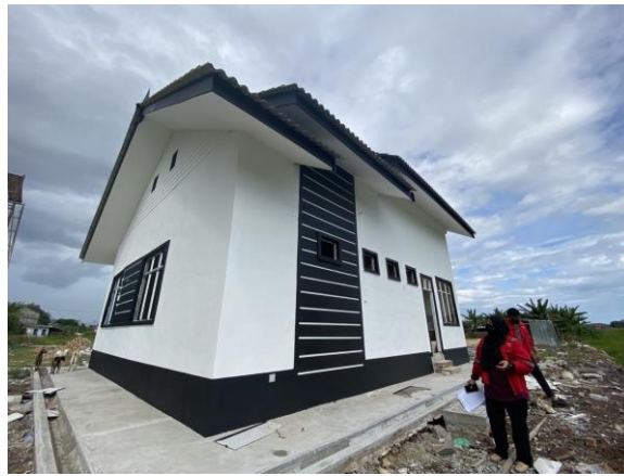
Figure 3.22 Check building insulation at site Durian Burung.
