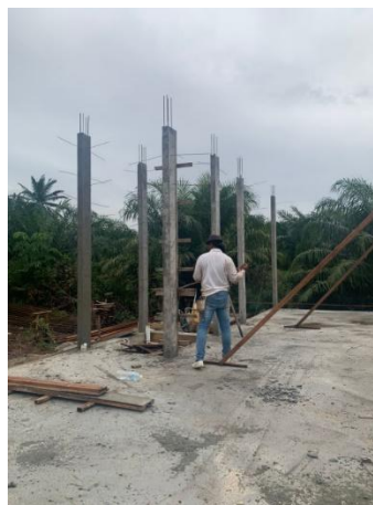
Figure 3.2.2 Process of cleaning the column and the floor
