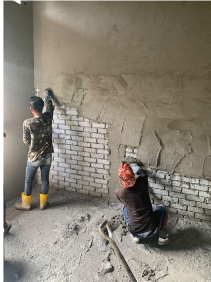
Figure 3.3.8 Process of plastering the entire wall of the houses.
