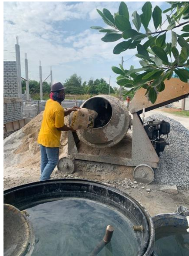
Figure 3.2.3 Mortar are being mixed with concrete mixer
