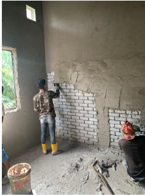
Figure 3.2.8(a): Plastering the wall for the finishes
