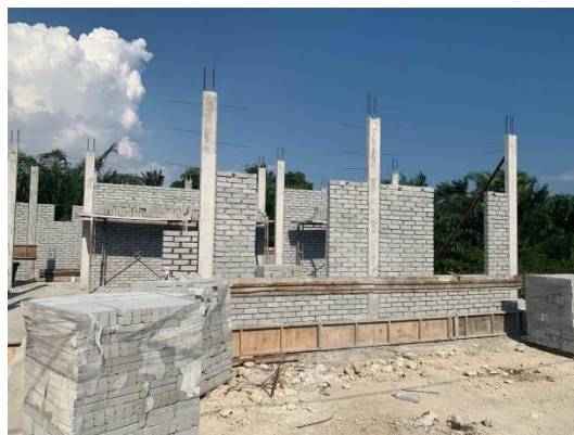
Figure 3.3.5 the wall part of the living room.
