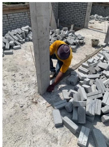
Figure 3.2.4 String that been tied between two column
