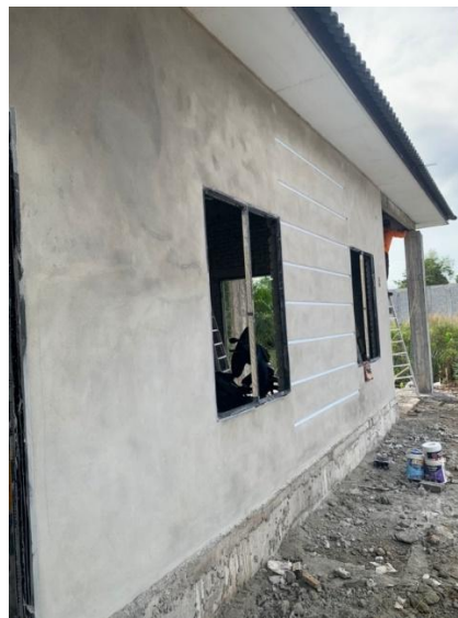
Figure 3.2.8(b): The wall after plastering process
