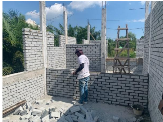
Figure 3.2.6 The bricklaying process of wall
