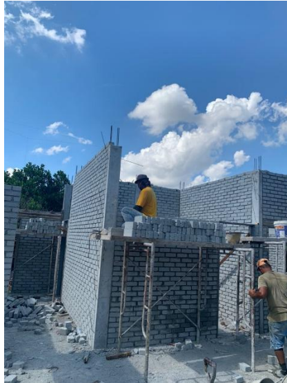
Figure 3.3.6 bricklaying process for internal wall of bedroom
