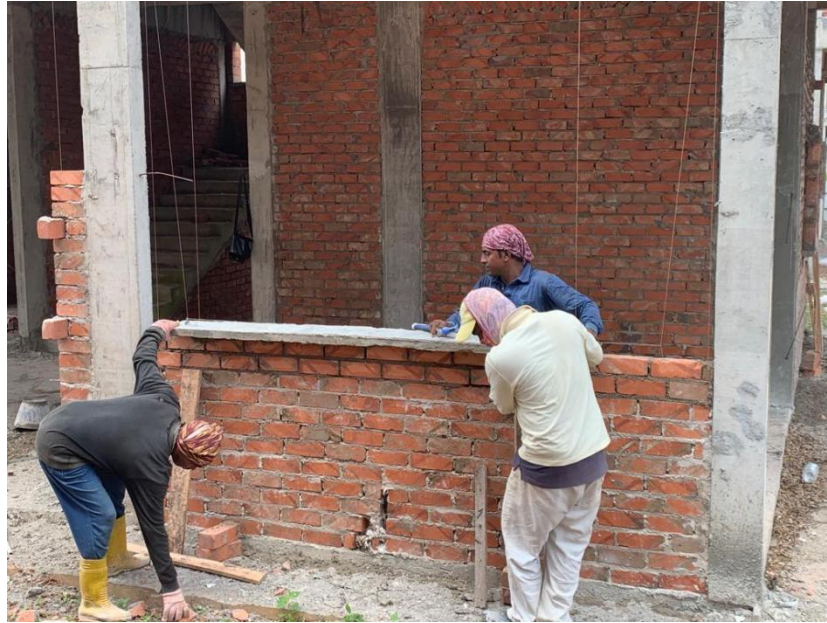
Figure 3.2.9: The window opening part of the wall.
