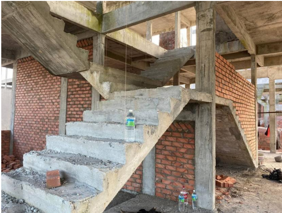
Figure 3.2.7: Bricklaying the wall process.
