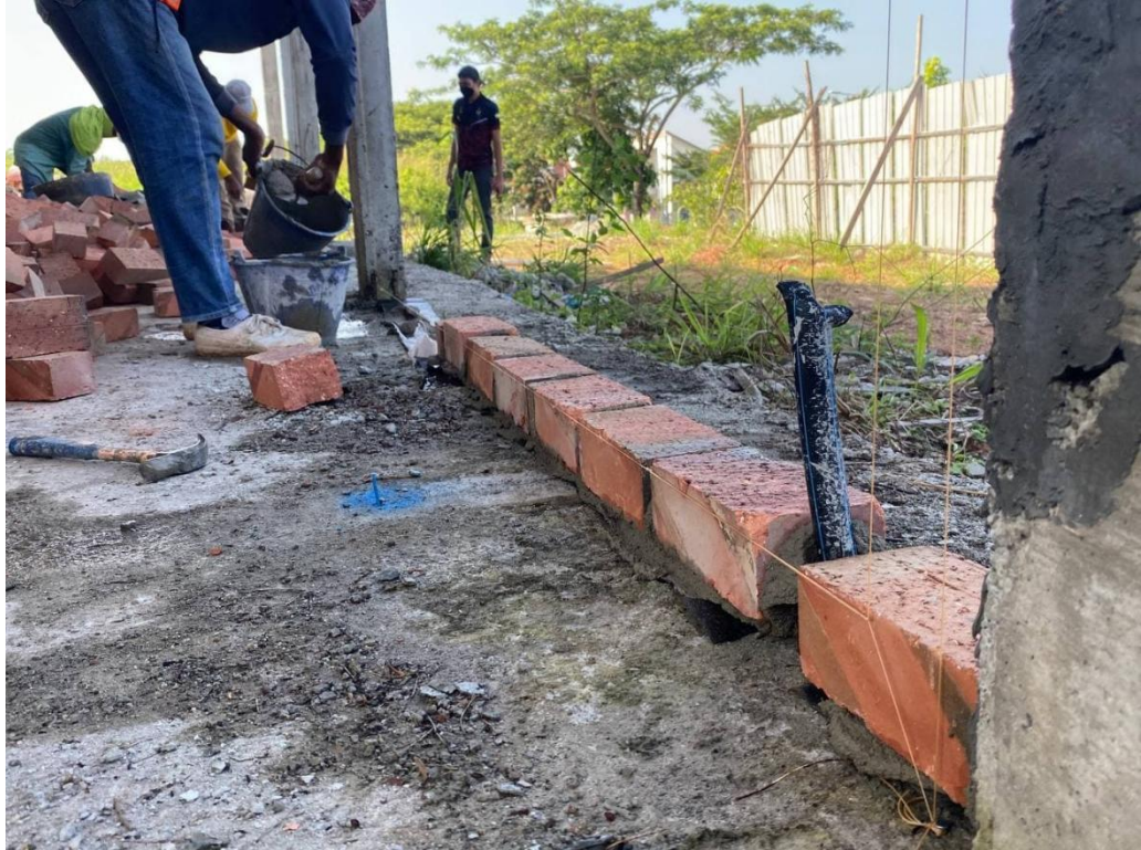
Figure 3.2.5: Strings that pinned together in between column.
