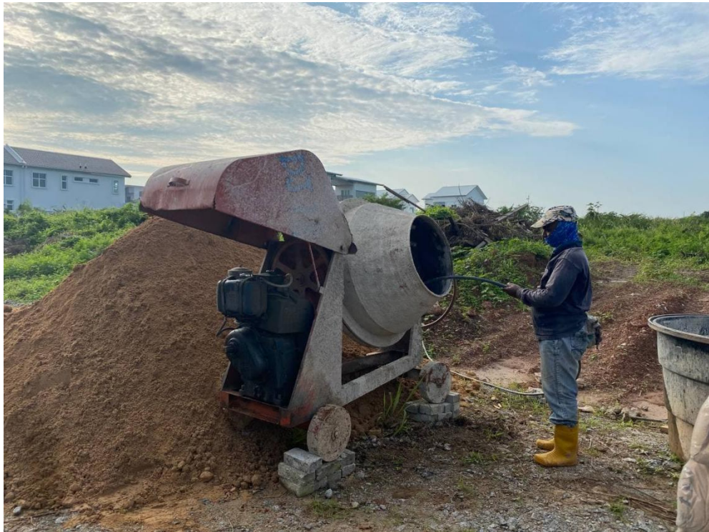
Figure 3.2.4: Mortar are mixed using the concrete mixer.
