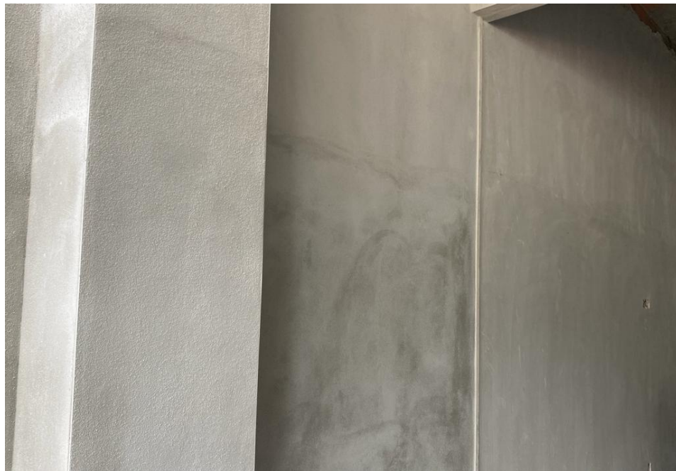
Figure 3.2.12: The wall after plastering process finish.
