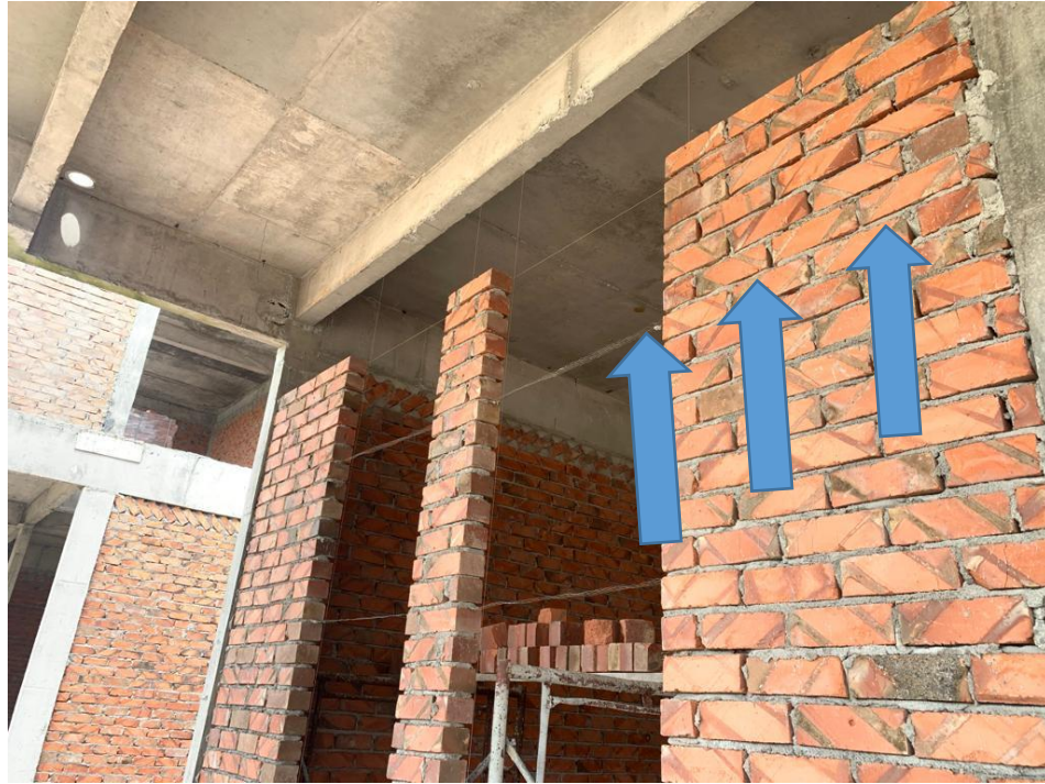
Figure 3.2.8: An exmet wire inside the layer of the brick wall.
