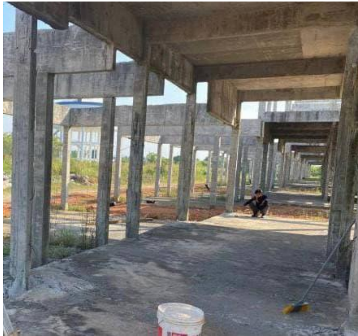
Figure 3.2.2: The floor of building that have been cleaned before bricklaying process.
