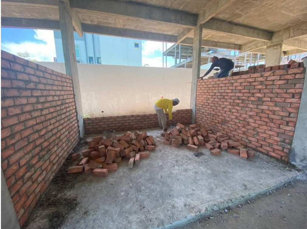
Figure 3.2.3: The clay brick that lifted from stock pile to the construction site.
