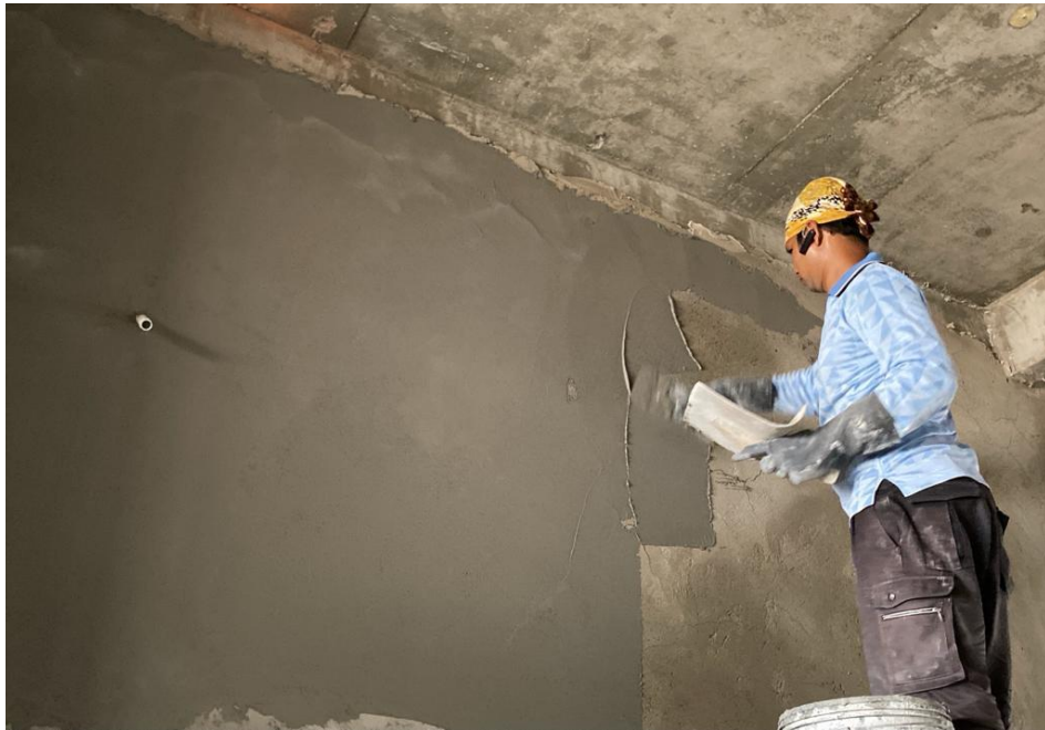
Figure 3.2.11: Plastering the top of wall for the finishes.
