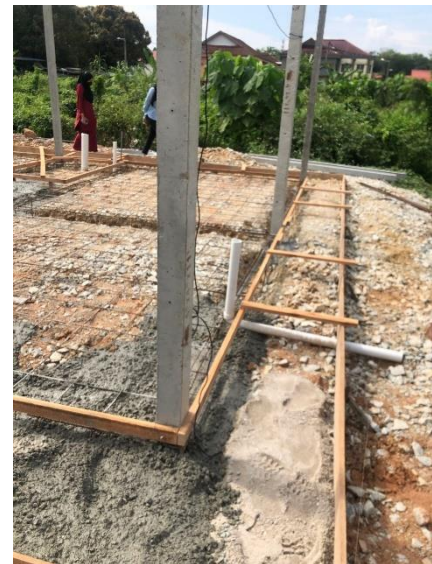
Figure 6: Installation ground beam at Sungai Buloh
