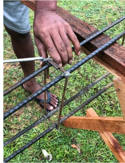
Figure 13: Installation of iron wire to ground beam rebar
