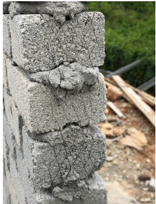
Figure 11: wire mesh provide every layer of sand brick
