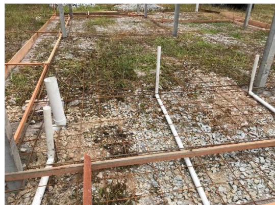
Figure 8:Installation of pipe before do the concrete
