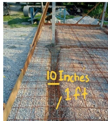
Figure 7: Depth and width of ground beam
