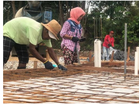
Figure 14: Jointing BRC using iron wire
