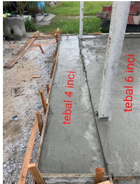
Figure 9: Slab and sidewalk formed after finish pour the ready mix concrete
