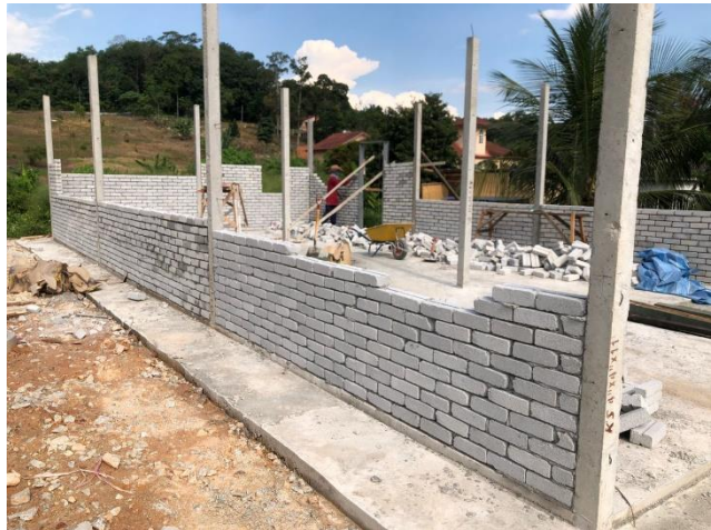
Figure 10: Installation of sand brick wall from pole to pole
