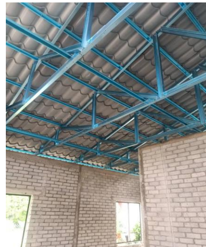
Figure 15: C channel iron and Batten iron are used for roofing work
