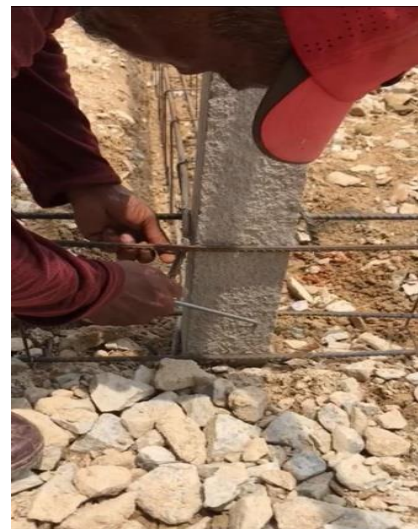
Figure 12: installing ground beam reinforcement bar with poles
