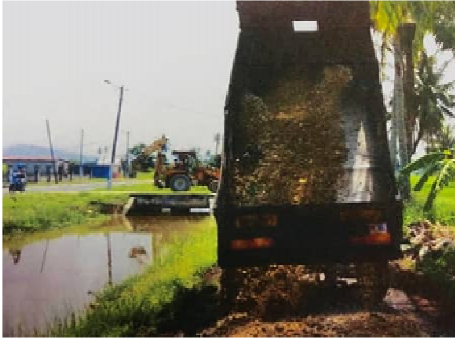
Figure 3.11: A lorry pour the crusher run on road
