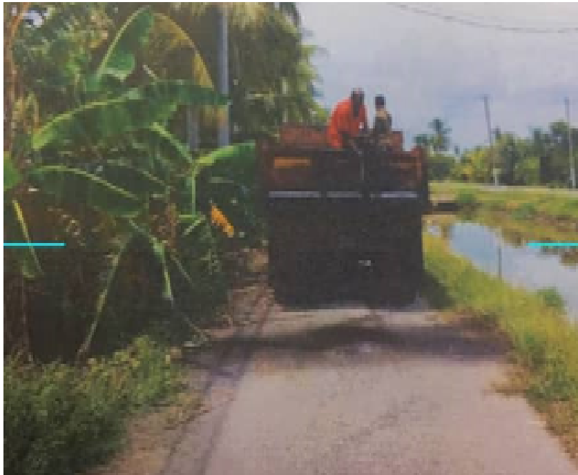
Figure 3.12: Worker spraying bitumen
