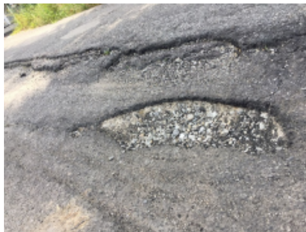
Figure 3.3: The pothole
