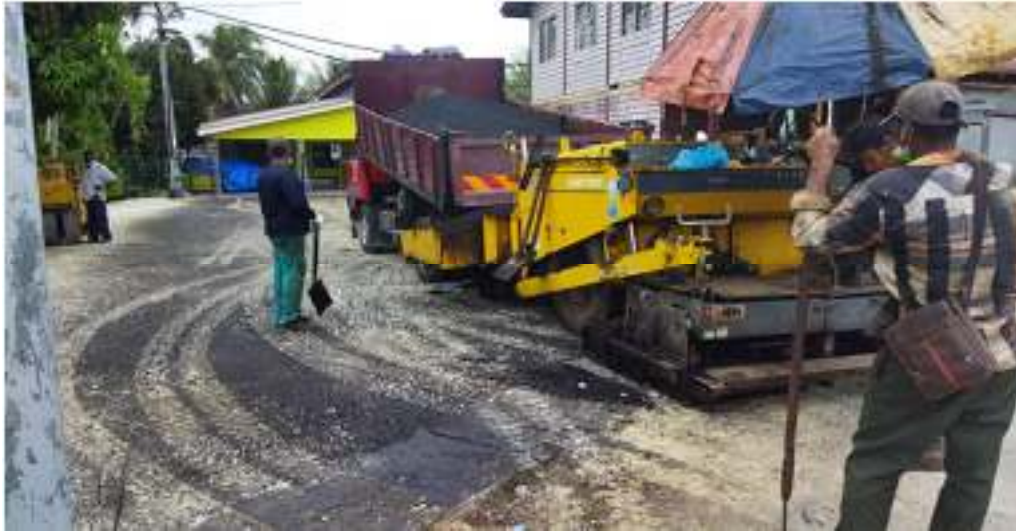
Figure 3.13: A lorry fill the paver with premix
