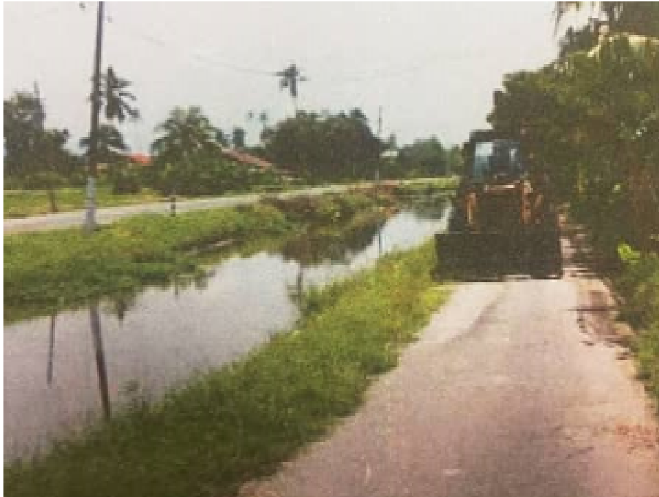
Figure 3.9: A backhoe cleaning the side road from grass
