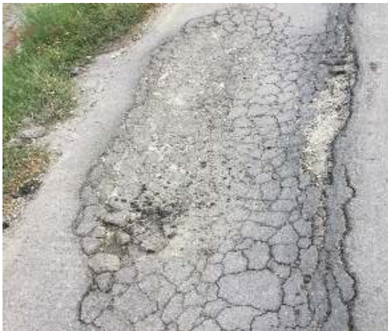
Figure 3.1: road cracking
