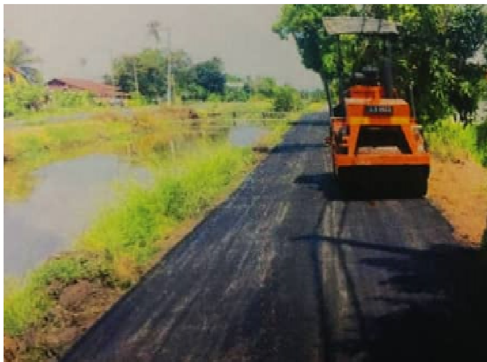
Figure 3.10: A roller compact the premix
