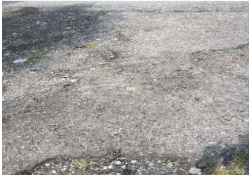
Figure 3.4: Road ravelling
