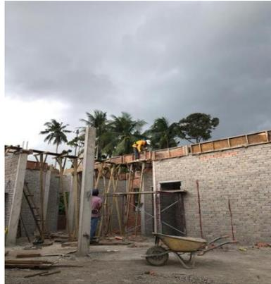
*Figure 27 : Preparing Beam formwork*
