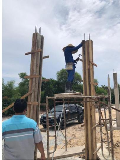
*Figure 12 Stripping of formwork*
