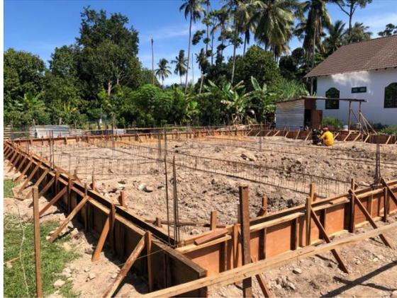
*Figure 19: placement of reinforcement and formwork installation*
