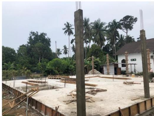
*Figure 26 : Concrete column construction process*
