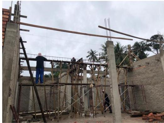
Figure 28 : Install reinforcement for the beam
