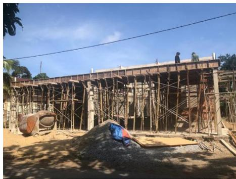
*Figure 33 : Formwork installment*
