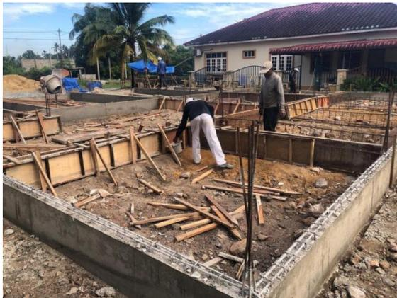
*Figure 20 : Removing the formwork*
