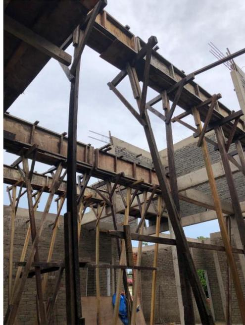
*Photos 15 Installation of formwork for roof beam*
