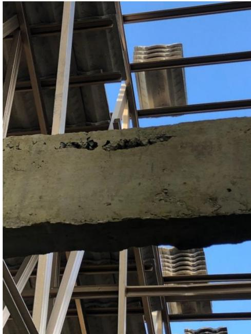
*Figure 37: Honeycomb defect*
