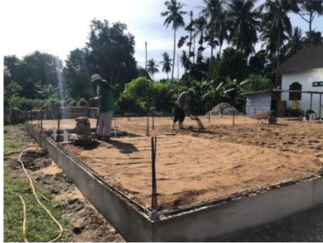
*Figure 22 : fill the space with the sand and use compactor machine*
