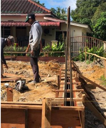
*Figure 14 Installation of beam*
