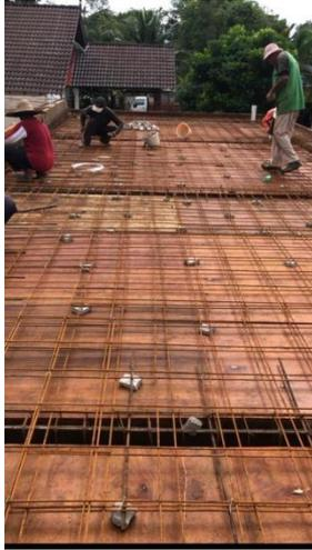
*Figure 17 Surface should be clean before concreting*
