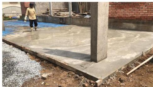
*Figure 31 : Concrete is cast on the reinforcement*
