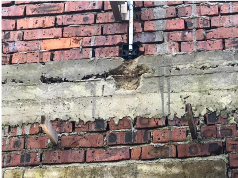
*Figure 38 Steel bar visible out from structure*
