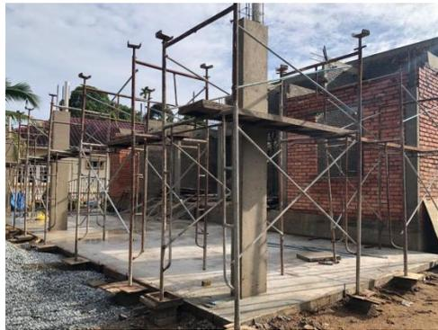
*Figure 32 : Staging scaffolding installment*
