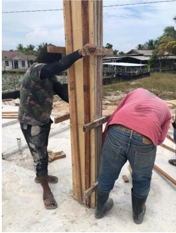
*Figure 10 Inspection the vertically before concreting*
