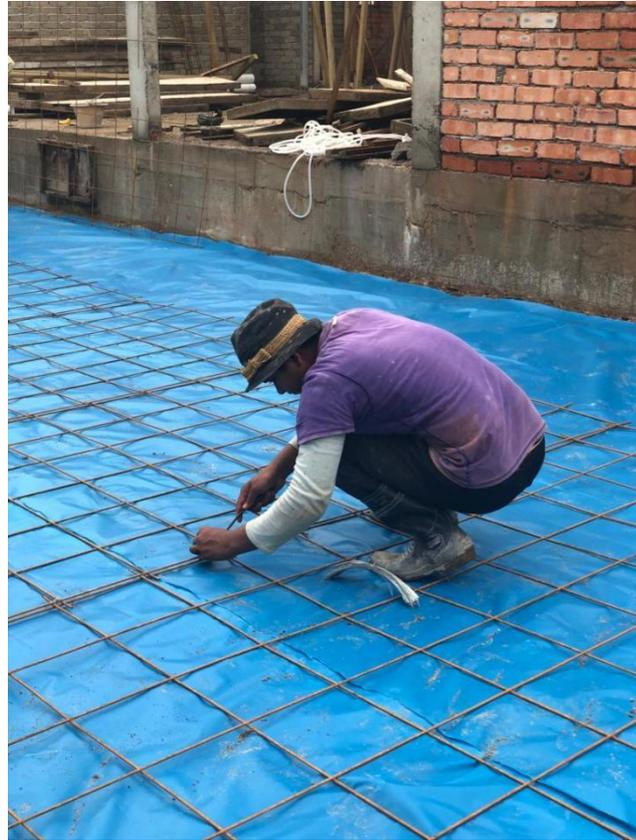
*Figure 7 Fixing the BRC*
