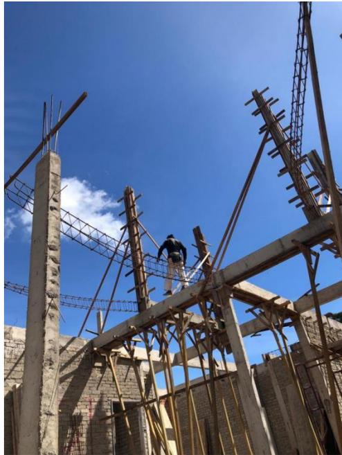
*Figure 13 Formwork of beam*
