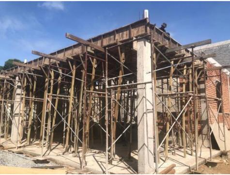
*Figure 18 the slab construction in progress*
