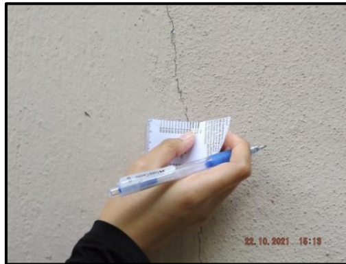
Figure 3.20 : Measuring The Defect Size
