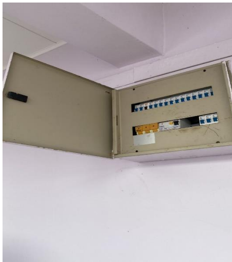
Figure 3.3.10: the steel plate on distribution box has been installed
