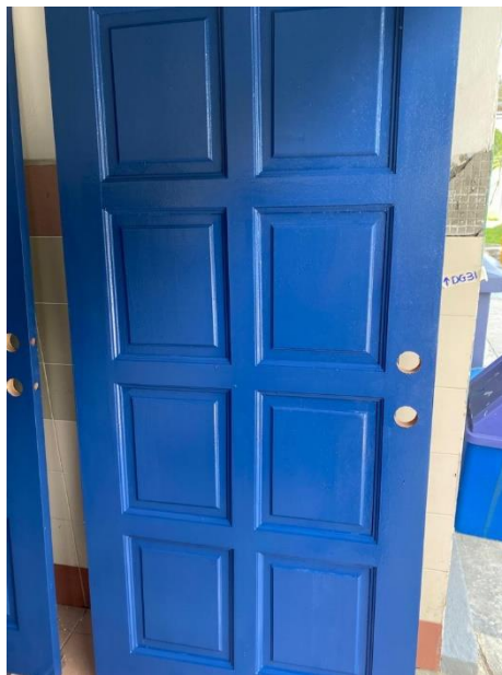
Figure3.3.7 : the door has been removed to do the maintenance
