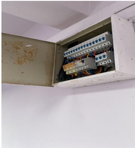
Figure 3.3.9 : the steel plate on distribution box is removed
