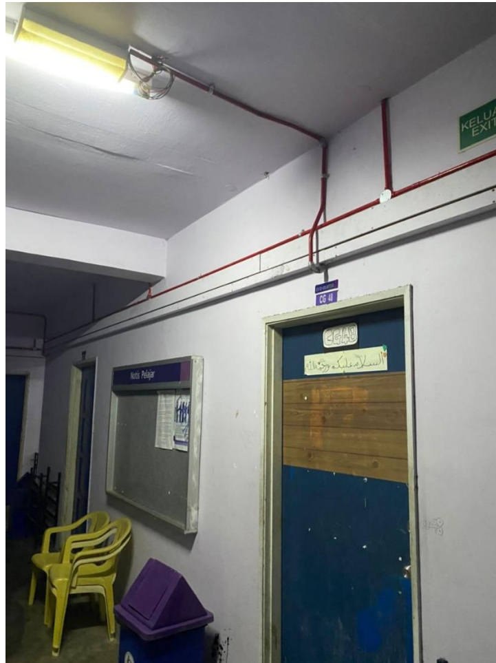
Figure 3.3.5: The steel panel has been installed and painted with white colour
