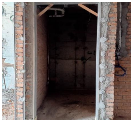
Figure 26: Brickwall for Study room at Unit 6
