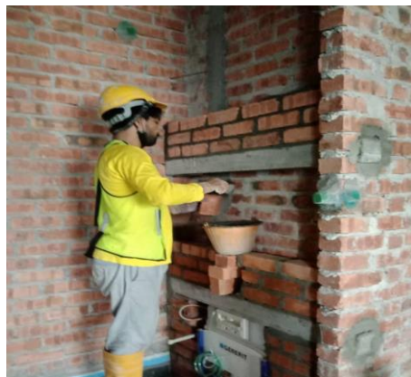
Figure 29: Brickwall process for WC low wall at Master bathroom
