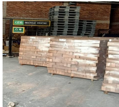
Figure 16: Cement and bricks stored in the shaded area
