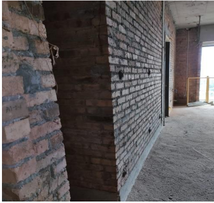
Figure 14: Brick wall at unit
