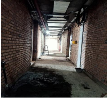
Figure 21: Brickwall for Main entrance from Corridor
