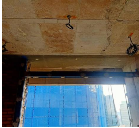
Figure 30: Brickwall process for lintel door opening
