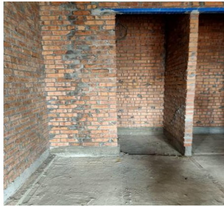
Figure 24: Brickwall for Master Bathroom
