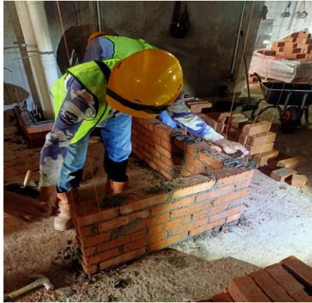
Figure 12: Provide exmet reinforcement on the bricks
