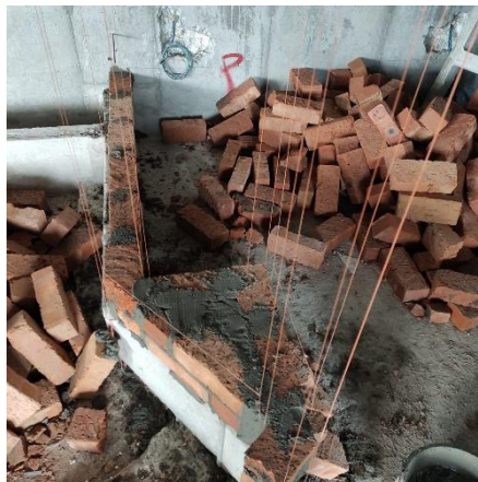
Figure 11: Laying brick
