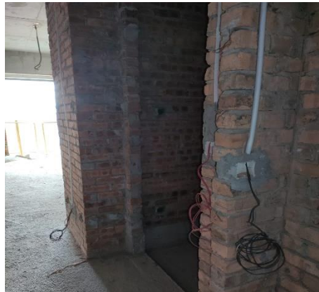
Figure 25: Brickwall for Powder room at Unit 3
