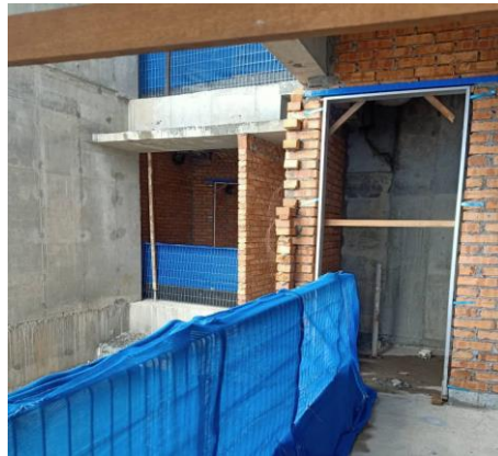
Figure 28: Brickwall for Bathroom 2 at Unit 4
