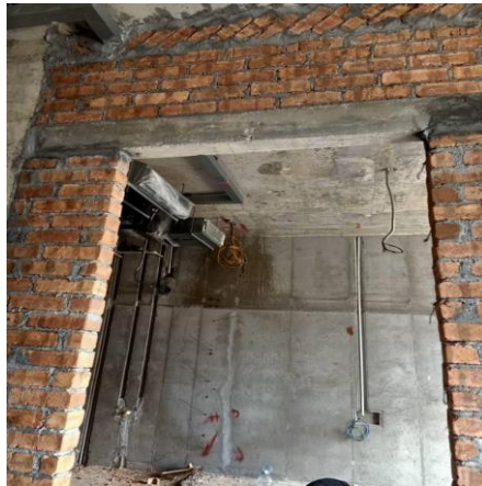
Figure 13: Lintel at door opening
