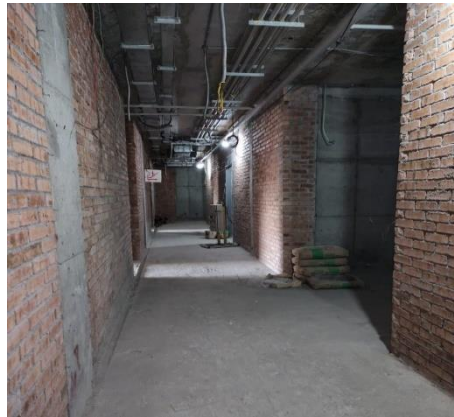
Figure 18: Brickwall for Corridor Level 24
