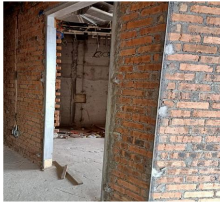
Figure 27: Brickwall for Bedroom 2 at Unit 11
