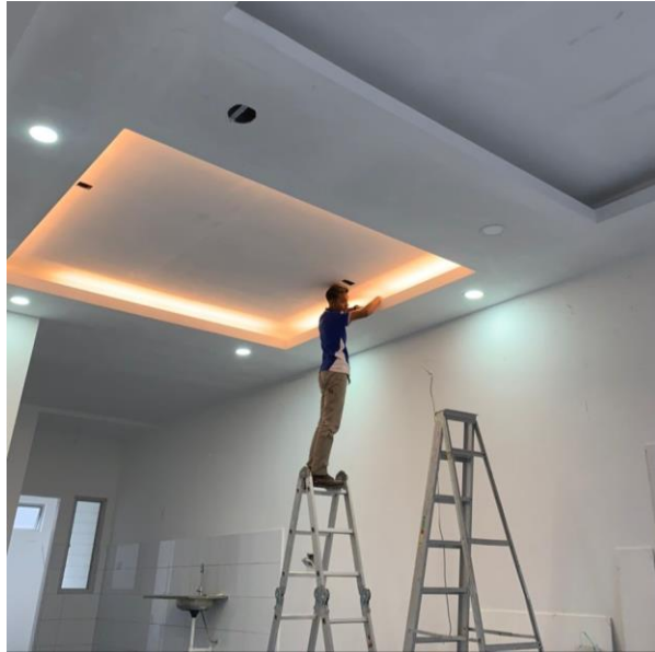
Figure 3.1: Finish product of lighting installation
