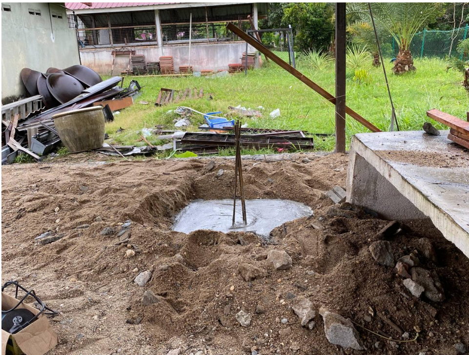
Photo 3.4 concrete pad foundation ,Kuala Lipis, Pahang
