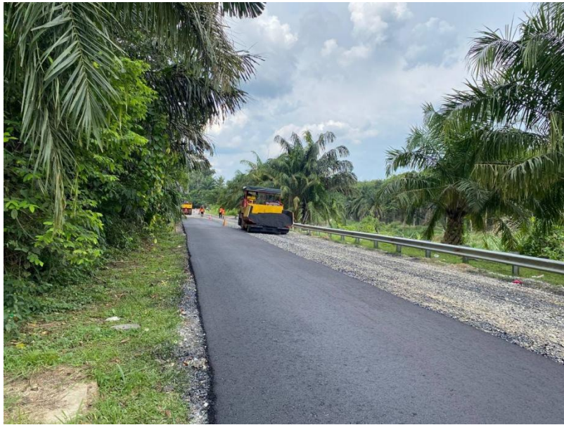
Photo 2.7 Jalan Besar Budu, Benta Estate
