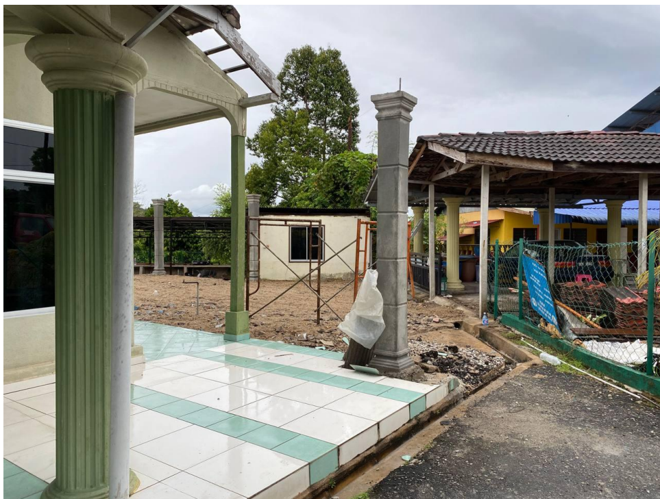
Photo 3.5 Concrete pillar , Kuala Lipis, Pahang
