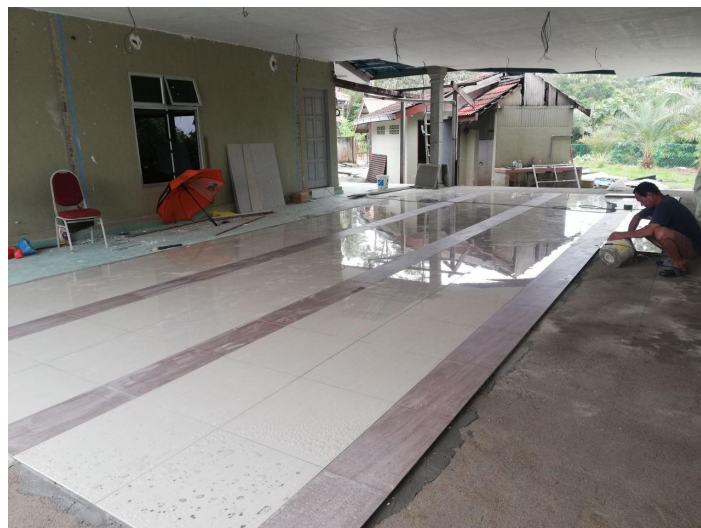
Photo 3.7 applying mortar to tiles , Kuala Lipis, Pahang
