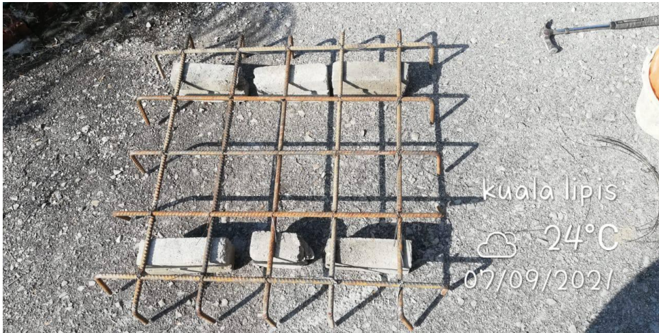
Photo 3.3 reinforcement bar pad footing ,Kuala Lipis, Pahang
