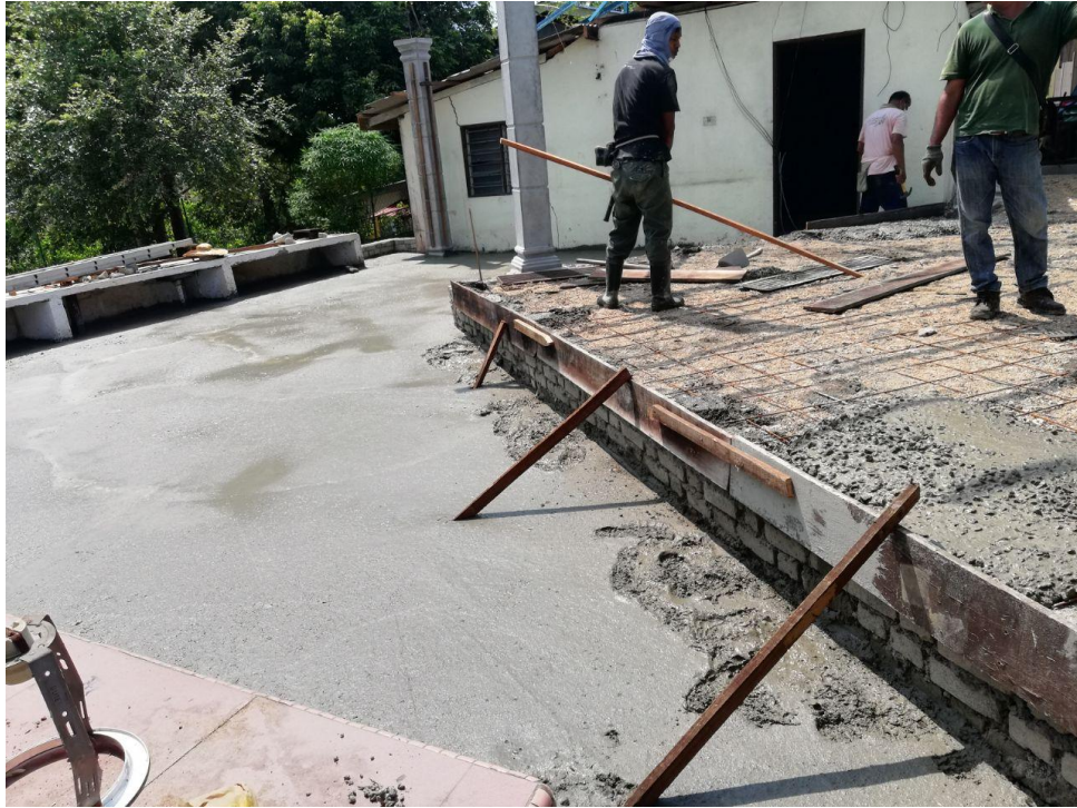
Photo 3. 6 concrete the slab, Kuala Lipis, Pahang
