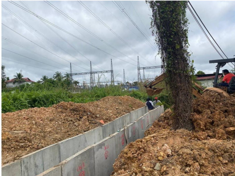
Photo 2.5 86% progress installation of culvert
