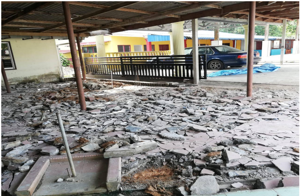
Photo 3.2 excavate the old tiles and soil, Kuala Lipis, Pahang
