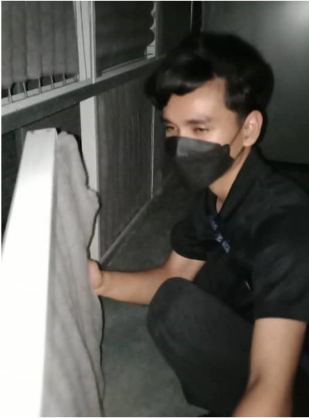
Photo 3.2.6: Reinstall air filters
