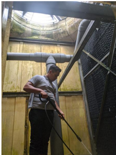
Photo 3.2.11: The inside of the cooling tower is cleaned and washed
