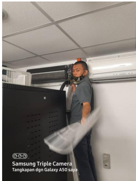
Photo 3.3.3: Remove air filter
