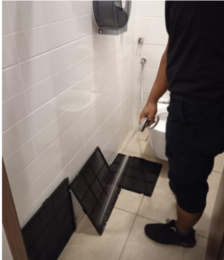
Photo 3.4.4: Wash the air filter with water
