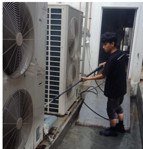
Photo 3.3.9: Clean the fin and body of the outdoor unit
