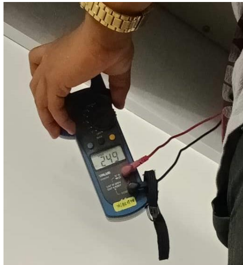
Photo 3.3.7: Check the voltage
