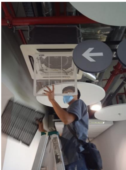
Photo 3.4.3: Uninstall the air filters
