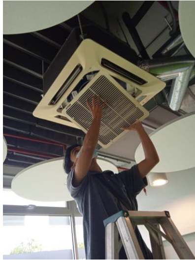
Photo 3.4.2: Open the front frame
