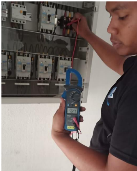
Photo 3.3.11 Check the voltage
