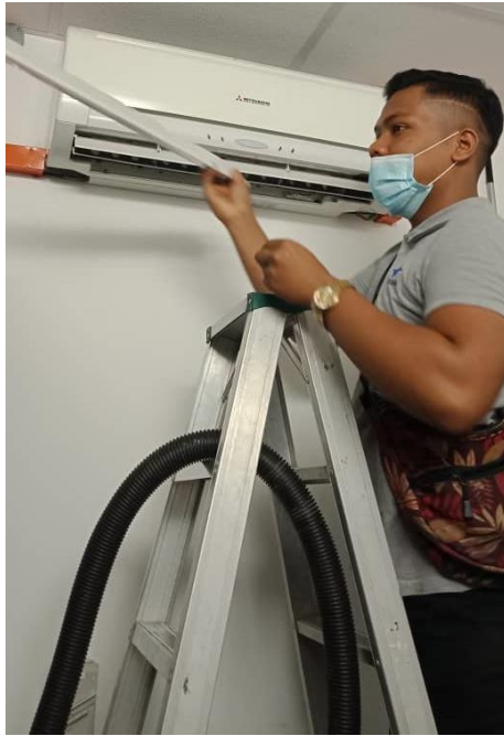
Photo 3.3.2: Open front panel of the indoor unit
