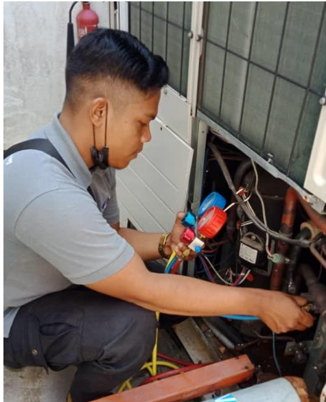
Photo 3.3.10: Check the quantity of the gasses
