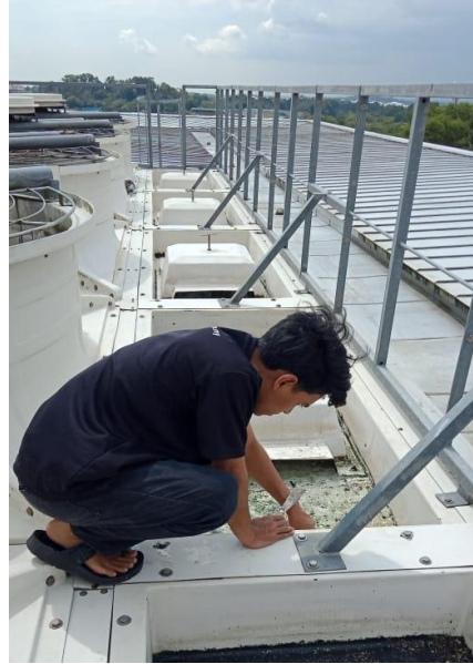
Photo 3.2.10: Cleaning the top of the cooling tower
