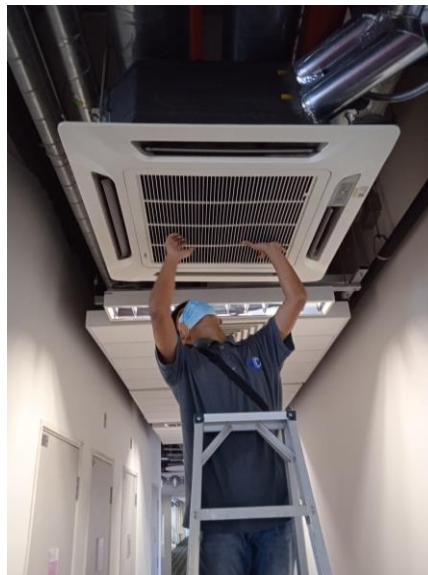
Photo 3.4.7: reinstall the filters and frame
