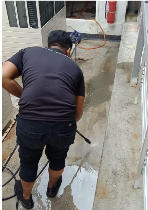
Photo 3.3.8: Cleaning the surrounding area
