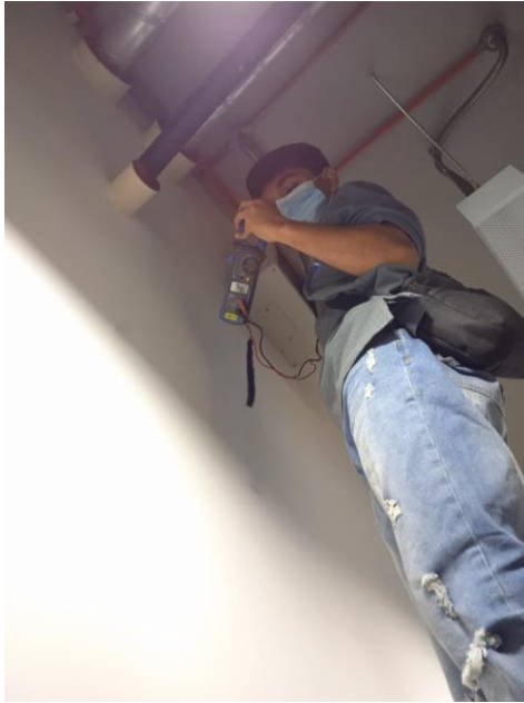
Photo 3.4.8: Check the voltage
