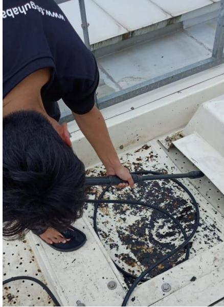
Photo 3.2.10: Cleaning the top of the cooling tower
