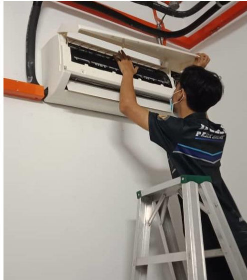
Photo 3.3.6: Reinstall the air filters
