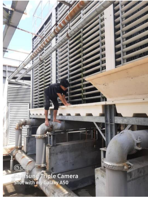
Photo 3.2.12: The outside of the cooling tower is cleaned and washed
