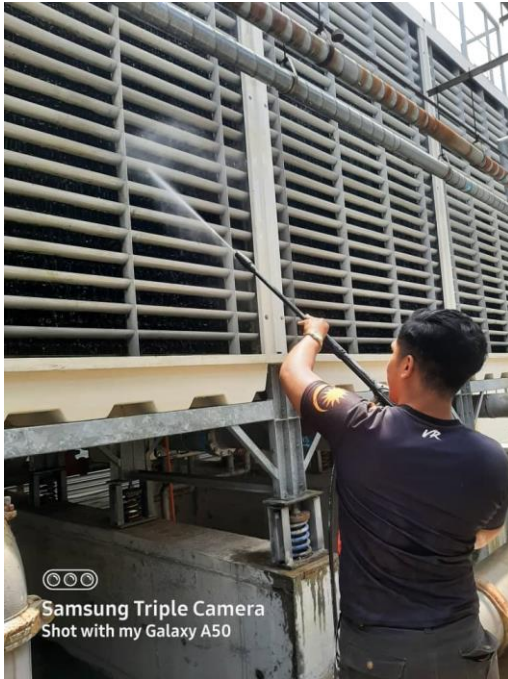
Photo 3.2.12: The outside of the cooling tower is cleaned and washed
