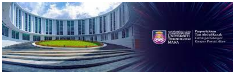
Figure 1: PTAR Campus Puncak Alam
