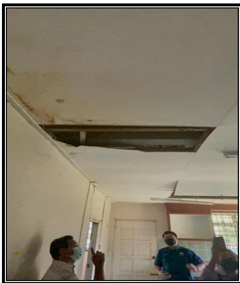
Figure 3.4: Broken ceilings
