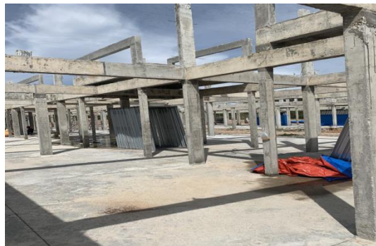
Figure 3.2.2: The floor has been cleared.
