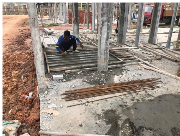
Figure 3.3.6: The mold has been poured into the mold box.
