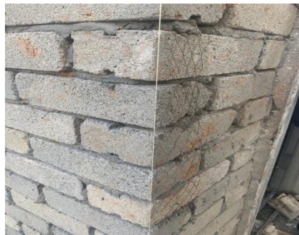
Figure 3.2.8: An exmet that has been installed.
