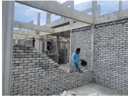
Figure 3.2.7: Workers are tying bricks.
