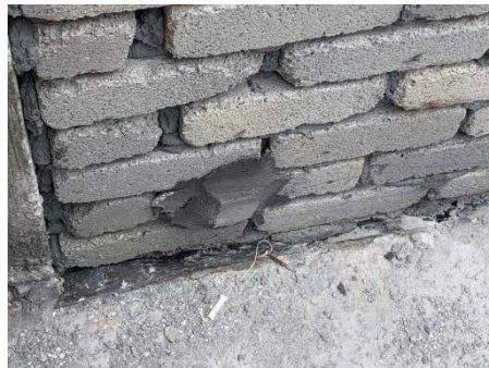
Figure 3.2.6: DPC that has been installed under the brick layer.
