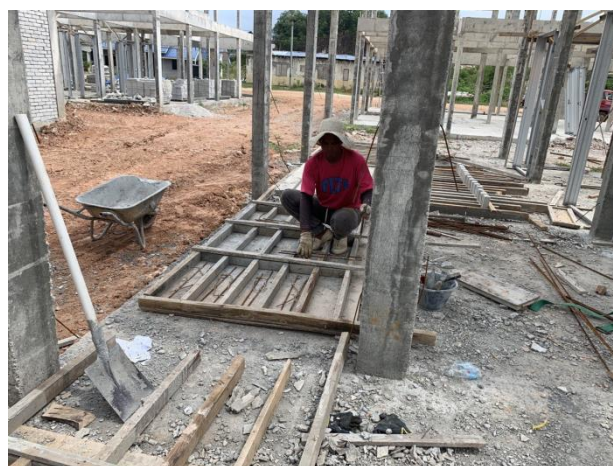
Figure 3.3.4 : Rebar was placed into the box.
