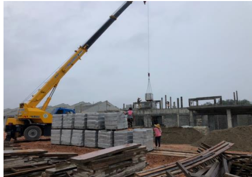
Figure 3.2.3: Bricks that have been lifted using a crane.
