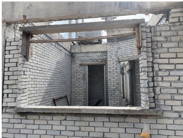
Figure 3.3.8: Lintel that has been installed.
