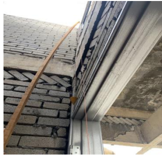
Figure 3.2.5: Using plumb bob to make the mark.
