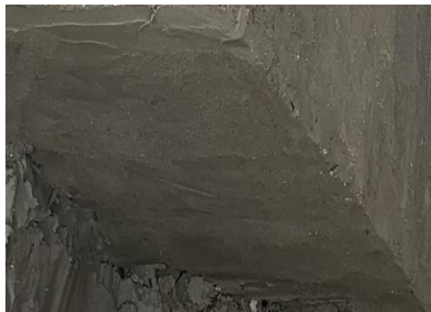
Figure 3.2.11: The walls have been plastered.
