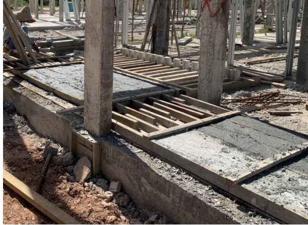
Figure 3.3.7: Lintel drying process.
