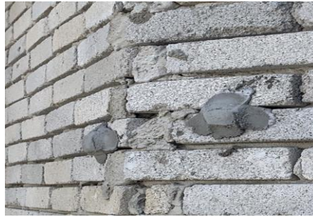
Figure 3.2.9: The walls have been marked for plaster.
