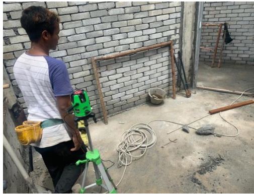
Figure 3.3.1: Measurements using laser levels.
