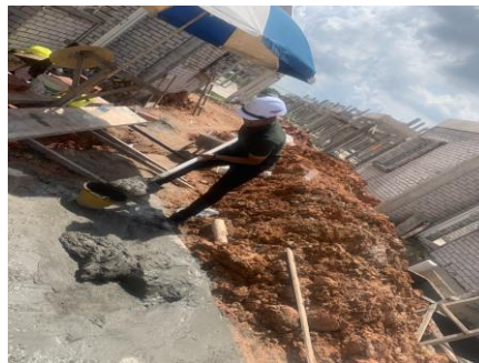
Figure 3.2.10: Mortar used for plaster.
