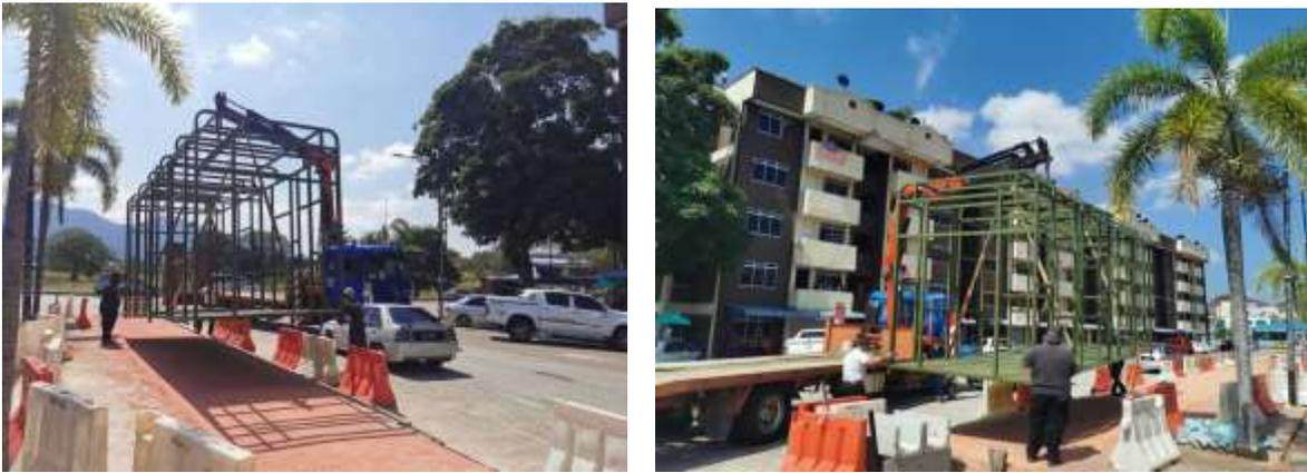
*Figure 3.5 : Lift up the frame structure using the crane to put on the slab*
