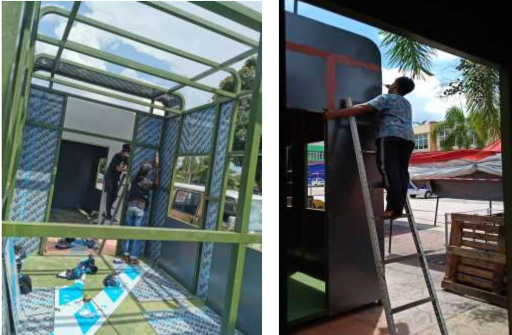
*Figure 3.6 : Frame structure connection works*
