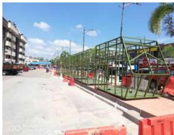
*Figure 3.4 : The frame structure is placed on top of the slab*
