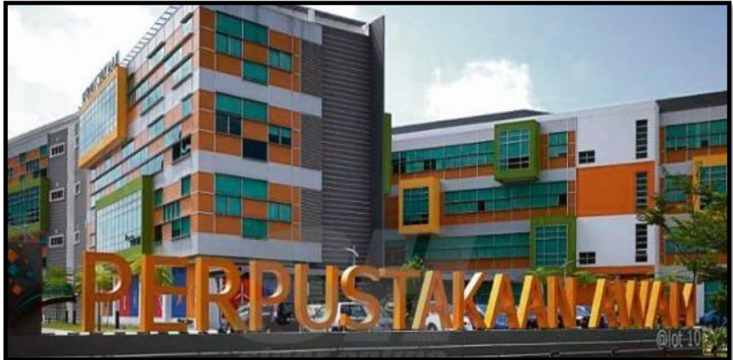
Figure 3: New building of PPAP
