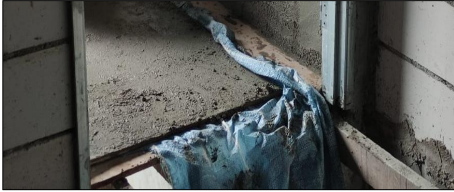
Figure 3.13: Canvas that has been used to protect the floor.
