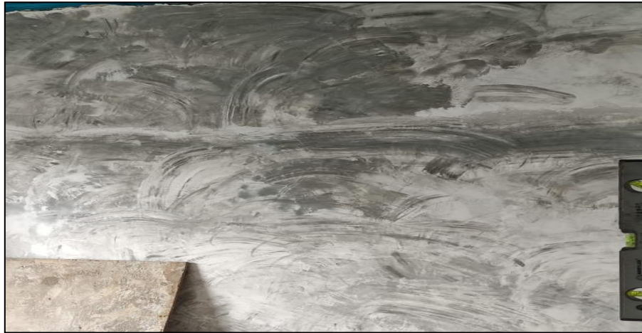
Figure 3.17: The result of the whole wall plastering work
