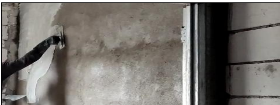
Figure 3.16: The first coat of lime plaster was being applied.
