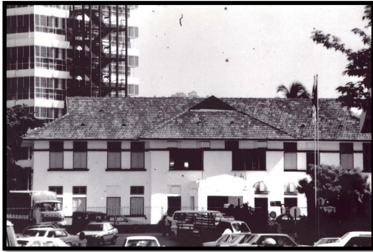
Figure 66: Old Rest House
