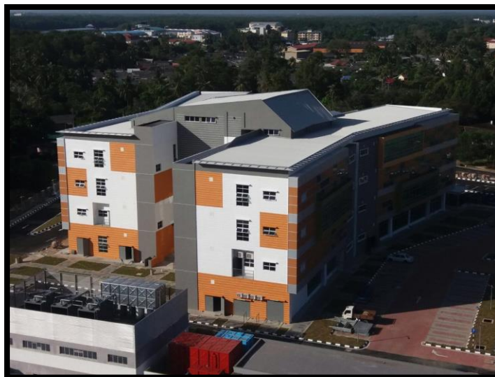
Figure 2: PPAP building that has been ready
