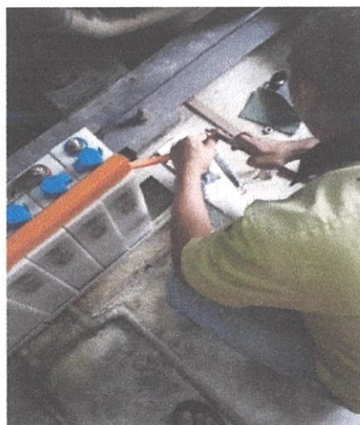
Photo 3.8: cutting cable wire
