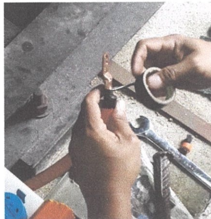
Photo 3.10: taping work
