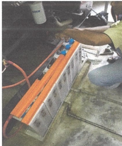
Photo 3.7: Remove cable from battery
