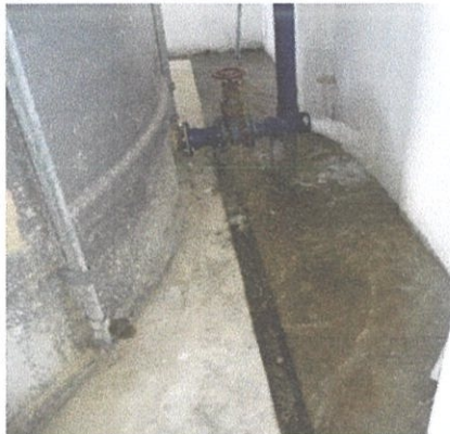
Photo 3.19: overflow pipe
