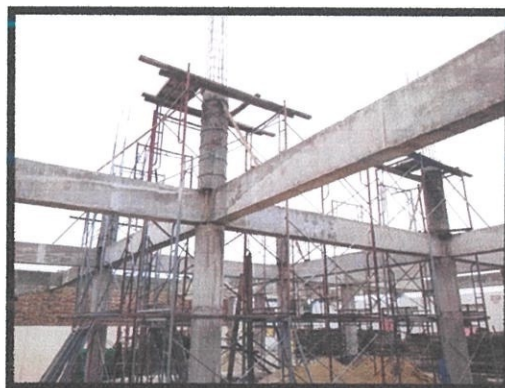
Photo 3.7: Support the formwork with bracing
