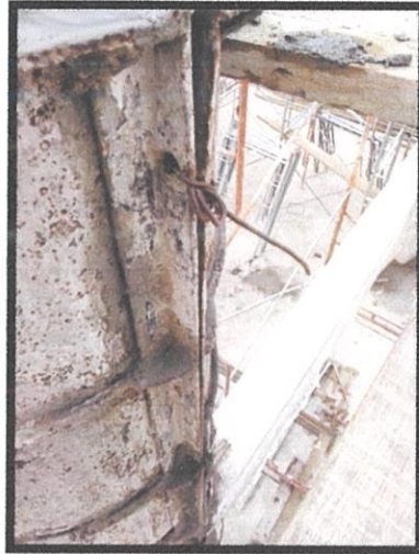
Photo 3.6: Tie using wires.
