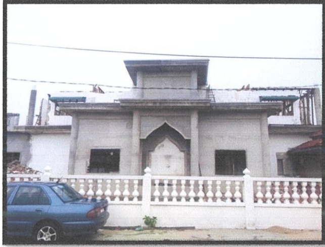
Photo 3.2: The rear elevation of building
