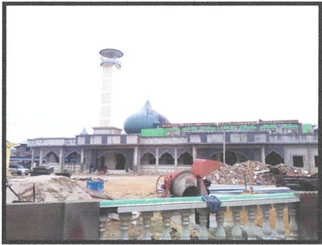
Photo 3.3: The right elevation of building
