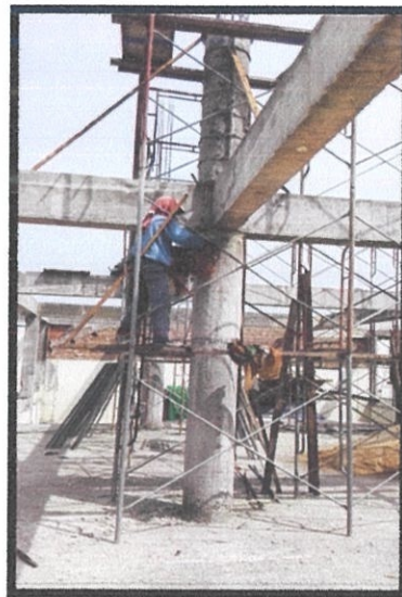
Photo 3.8: Cover the hole
