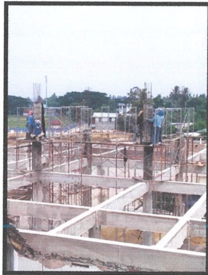
Photo 3.5: Installation of the formwork
