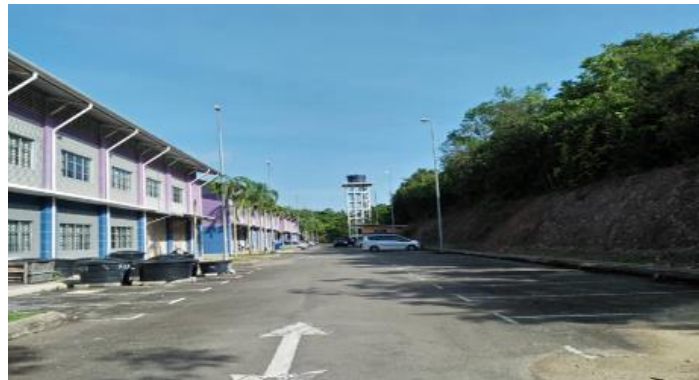
Admin Building (Site C)
