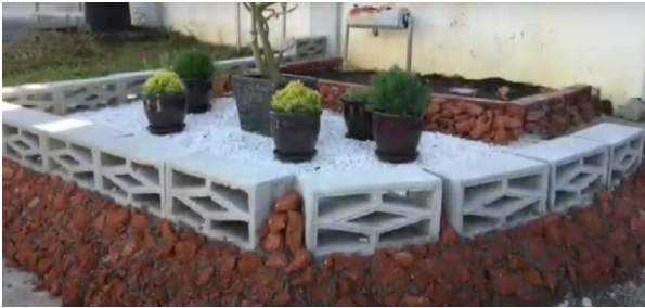
Figure 2: Landscape slope stabilization application using waste crush clay brick (WCCB)
