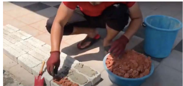
Figure 4: Application process of waste crush clay bricks on cement brick
