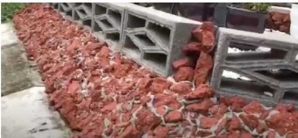
Figure 3: Application mixture between waste crush clay brick (WCCB) with cement glue
