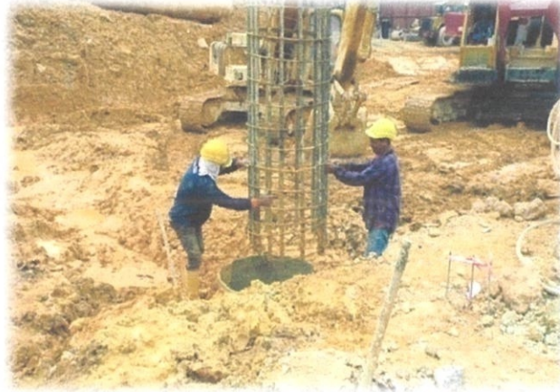
Photo 3.11: The installation of rebar cage in the bored hole.
