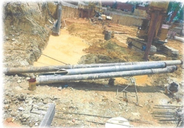
Photo 3.18: Tremie pipe in bored pile construction
