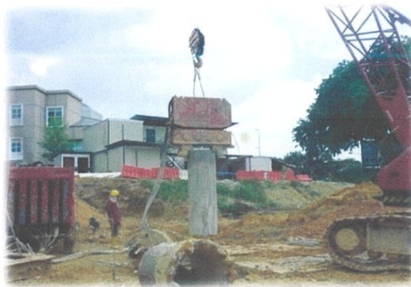
Photo 3.16: Steel casing installation by vibro hammer
