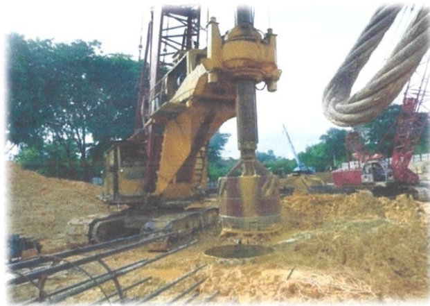
Photo 3.10: Drilling process using boring bucket.
