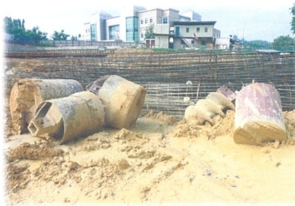
Photo 3.14: Auger and bucket used in bored pile construction.
