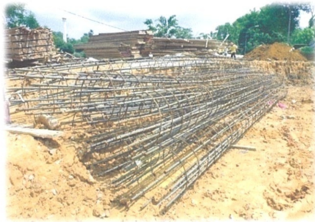
Photo 3.17: Reinforcement bar cage ready to be installed in the bore hole
