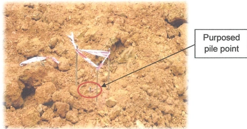
Photo 3.7: Steel pins around the purposed pile point.
