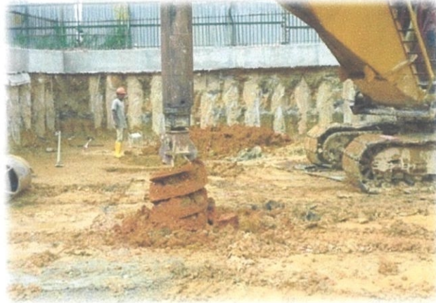
Photo 3.8: Remove the unwanted soil by drilling using soil auger.
