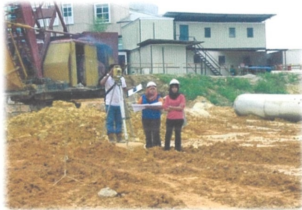
Photo 3.6: Surveyor peg out the pile point.
