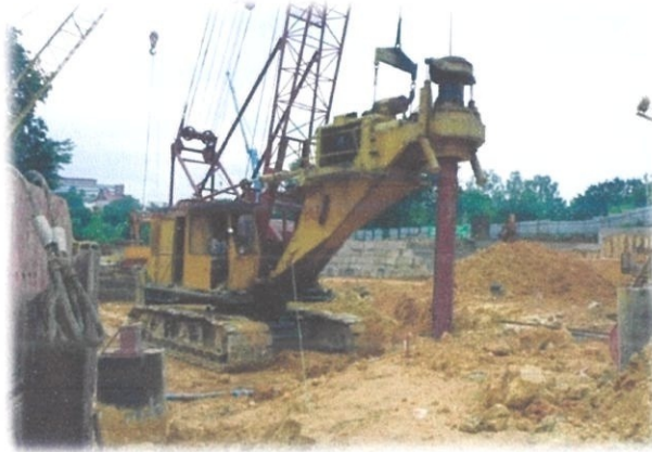
Photo 3.13: Drilling work by boring machine.
