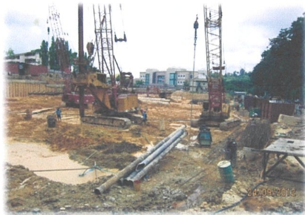
Photo 3.4: Current site condition.
