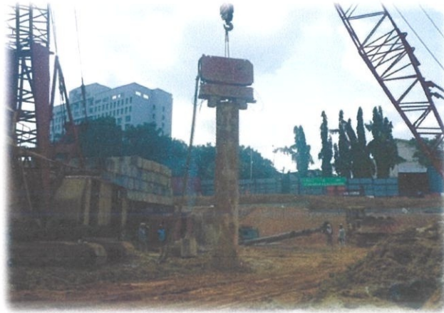
Photo 3.9: The installation of steel casing using vibro-hammer.
