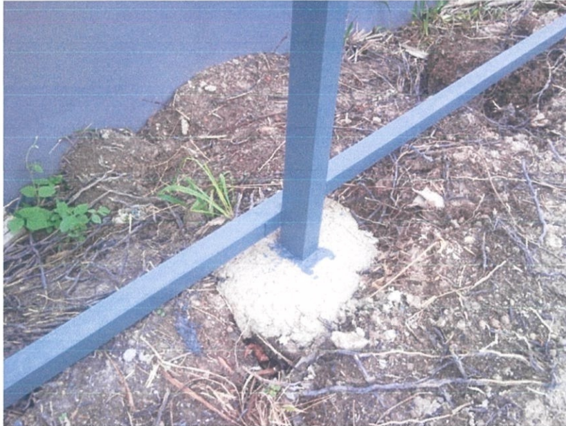
Photo 3.0 19 Frame of temporary Hoarding
