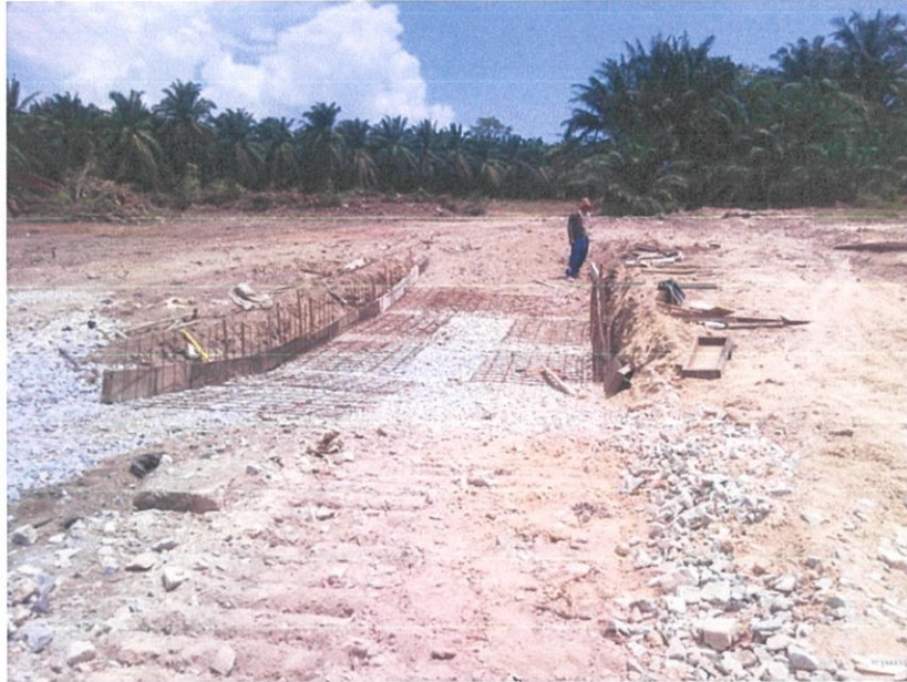
Photo 3.0 15 Washing Bay are install reinforcement and formwork
