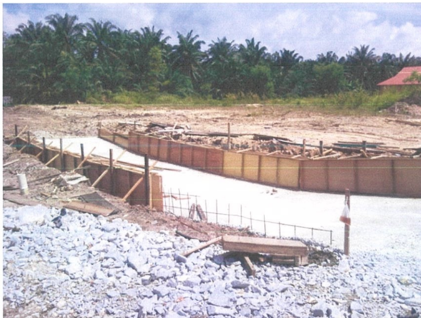
Photo 3.0 16 Washing bay are install formwork and concrete
