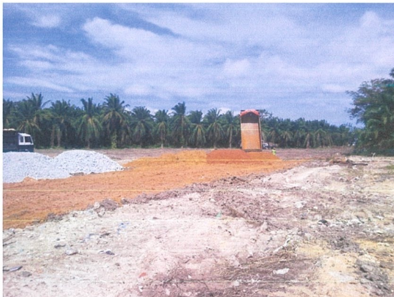
Photo 3.0 23 Stripping Topsoil Excavation
