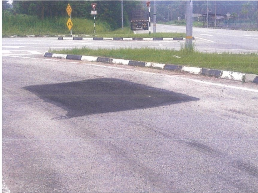
Photo 3.0 36 Road was repaired by put the new premix
