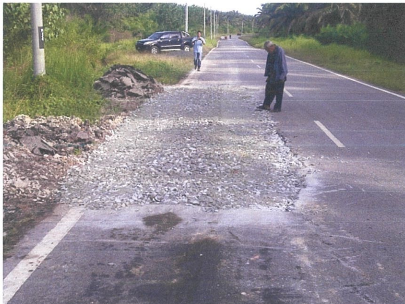
Photo 3.0 37 Road was repaired by put crusher run
