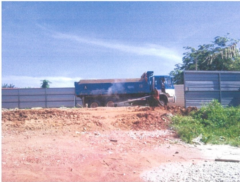
Photo 3.0 34 Tyre of the Lorries are washing with water jet
