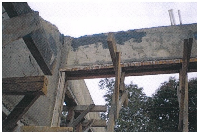
Photo 3.34: Honeycombis there on the concrete.
