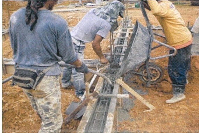
Photo 3.25: Process of pouring concrete on the ground beam at construction site.
