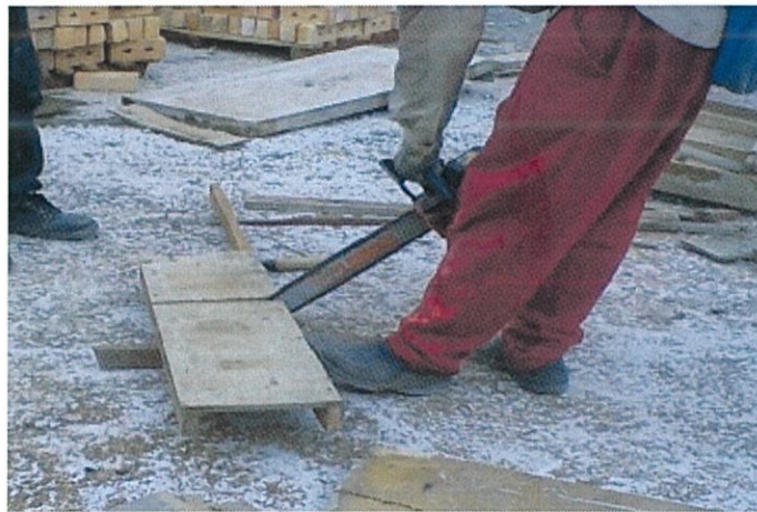
Photo 3.3: Worker cuts formwork with handsaw machine.
