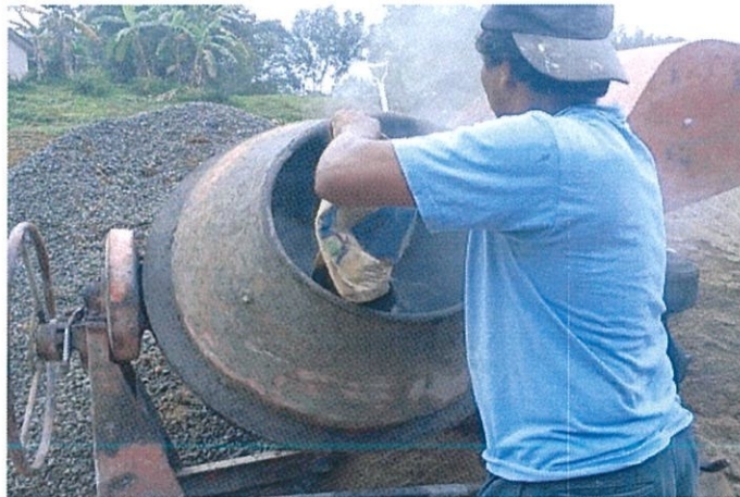
Photo 3.23: Mixing of concrete
