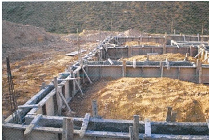
Photo 3.30: Concrete curing work left for 1-4 days at the construction site.
