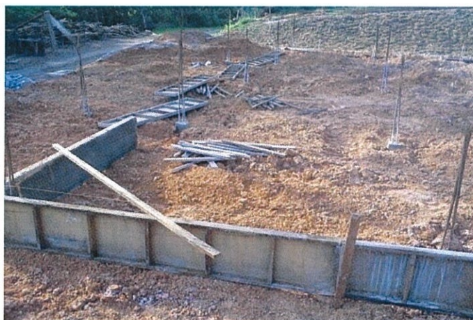
Photo 3.8: Installation formwork on the ground beam
