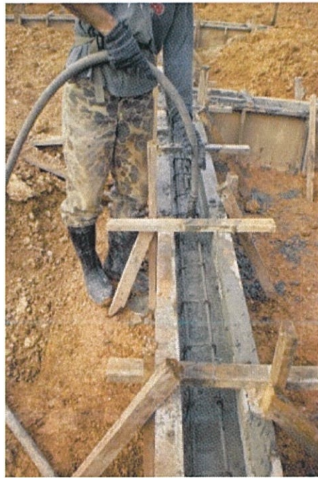
Picture 3.27: Compaction work done after the concrete put in a formwork using the poker vibrator machine.
