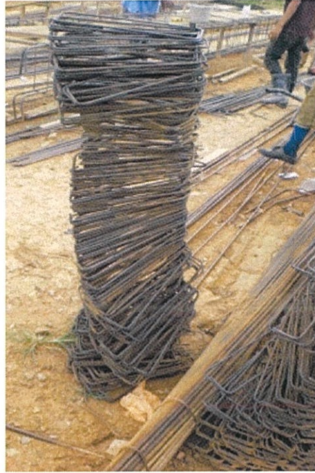
Photo 3.16: Steel bars which were bent at construction site.
