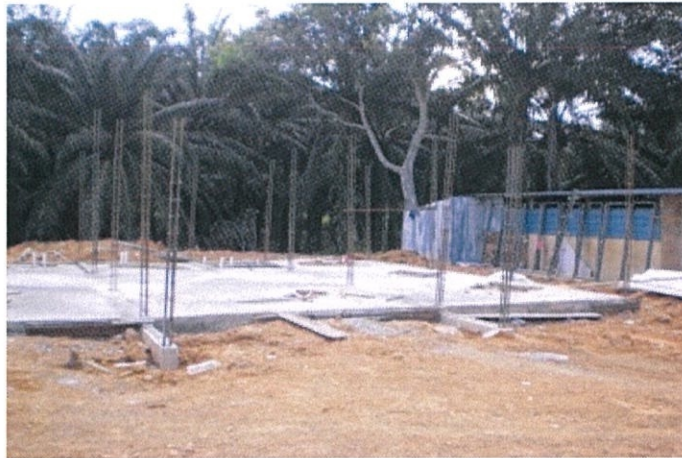
Photo 3.20: The installation of reinforcement on column at construction site
