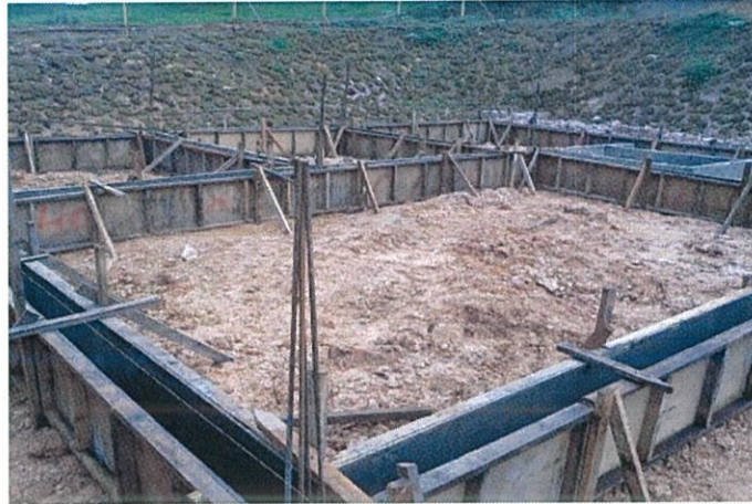
Photo 3.9: Formwork was complete on the ground beam
