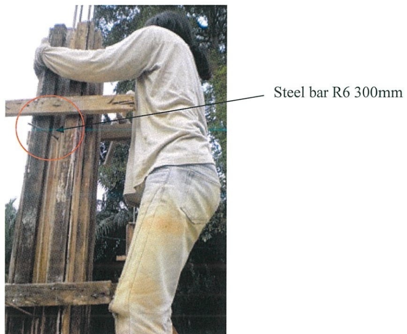
Photo 3.11: R6 300mm steel bar on the column
