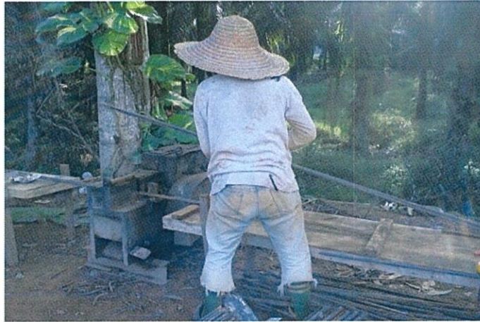
Photo 3.14: Steel bar cutting using steel cutter machine.
