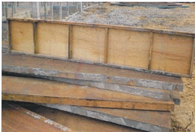
Photo3.6: Completed formwork at construction site.
