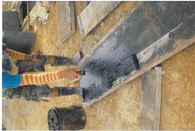
Photo 3.7: Paint black oil on the formwork
