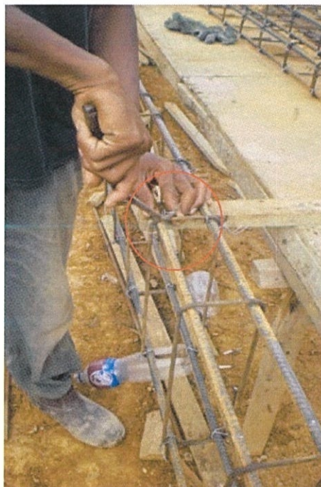
Photo 3.18: Slash Ring Bond that connects Y12 steel bars (horizontal) and R6 steel bar (vertical).
