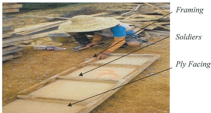
Photo 3.2: The parts of the formwork
