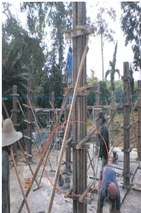
Photo 3.33: Flow out through the cracks of concrete formwork.
