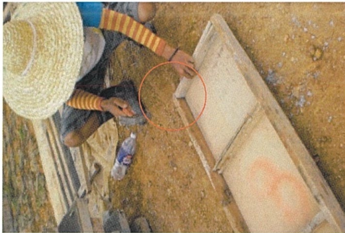
Photo 3.5: Nailing work on formwork.
