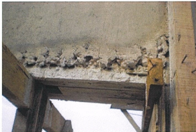
Photo 3.34: Honeycombis there on the concrete.
