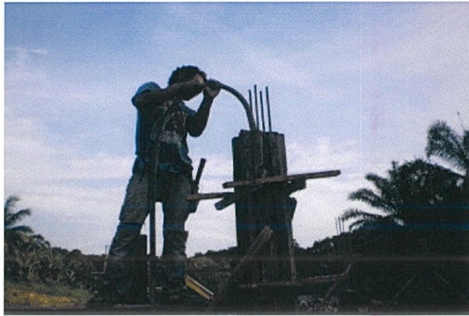
Photo 3.28: Compacting work on column
