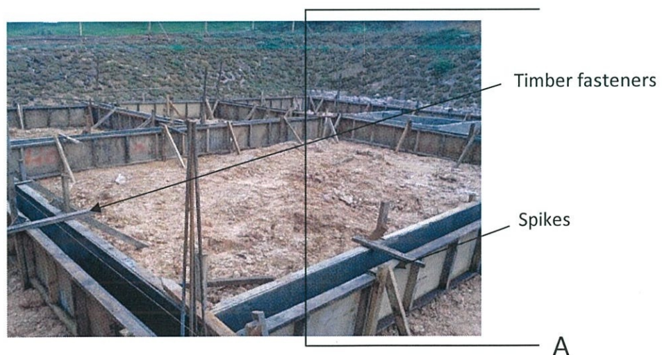
Photo 3.10: Timber fasteners and spikes on ground beam and section A-A
