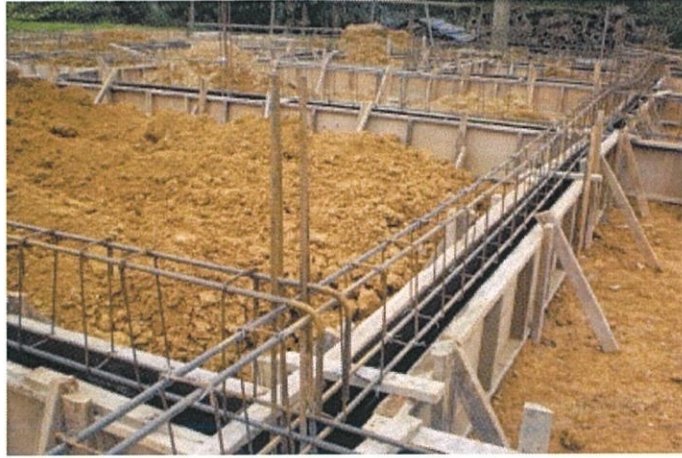
Photo 3.19: The installation of reinforcement on ground beam at construction site.
