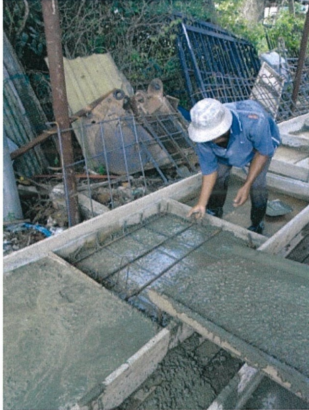
Figure 3.19 Application of RC bars on lean concrete
