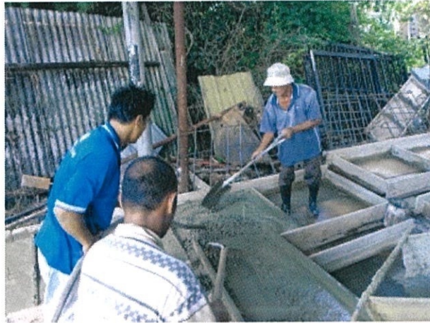
Figure 3.20 Formwork is fully filled with concrete
