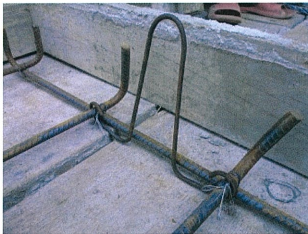
Figure 3.12 Hook is applied and binded with the RC bars
