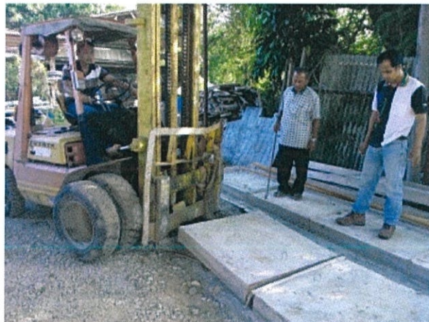
Figure 3.26 Lifting works for the separation of formwork underneath
