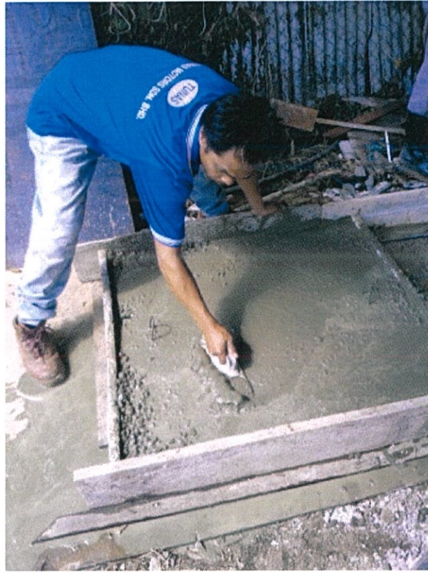
Figure 3.22 Plastering works on the concrete surface
