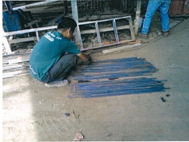
Figure 3.7 Placement of RC bars
