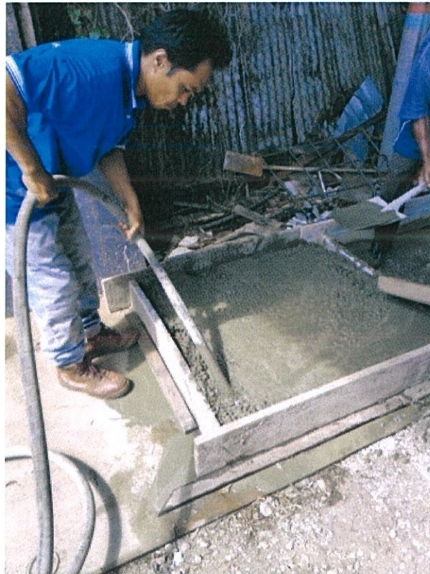
Figure 3.21 Vibration process of the concrete
