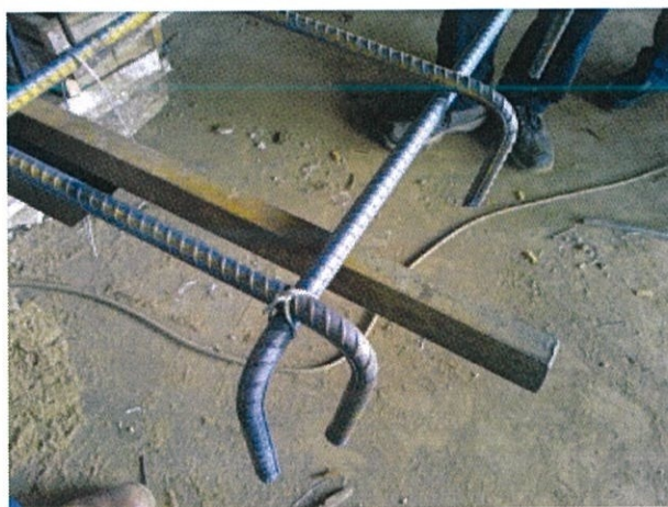
Figure 3.9 Picture of binded reinforcement bars
