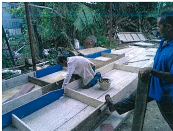
Figure 3.10 Formwork construction using plywoods
