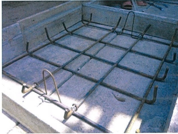
Figure 3.13 Binded hooks with RC bars
