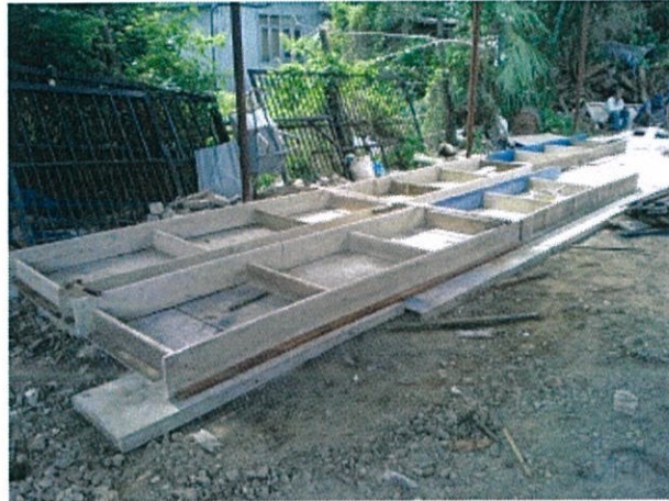
Figure 3.15 RC bars are removed from the formwork
