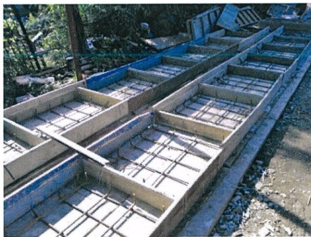
Figure 3.11 Placement of binded RC bars in formworks
