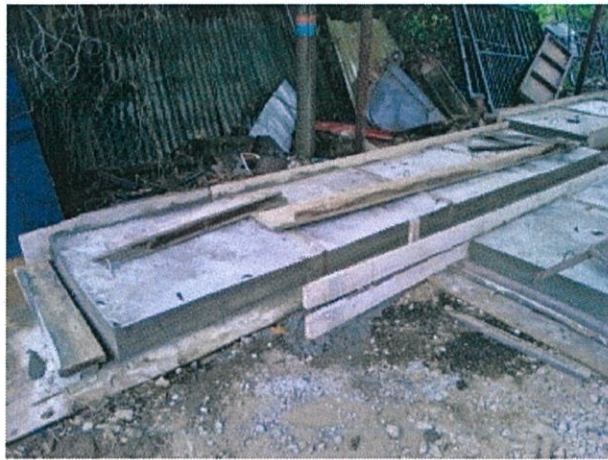
Figure 3.25 Removal of formwork from the drain closure
