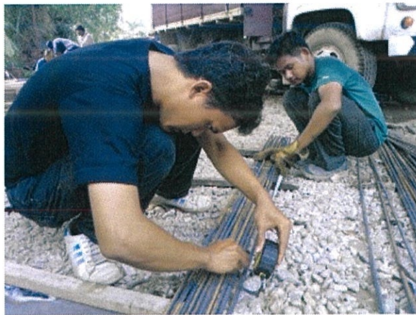
Figure 3.5 Marking process of 15m-long RC bars
