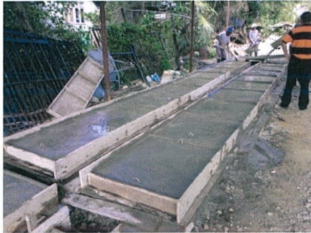
Figure 3.23 Concrete is dried for a week
