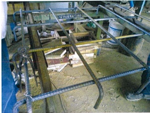
Figure 3.4 Picture of a binded reinforcement bars
