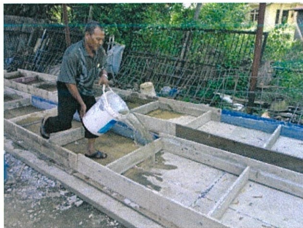
Figure 3.16 Formworks are moisturized using water
