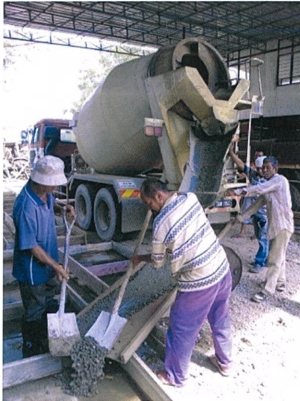
Figure 3.18 Concrete pouring process is carried out
