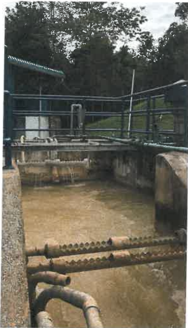
Figure 4.5 : The entrance of raw water from Kinta River
