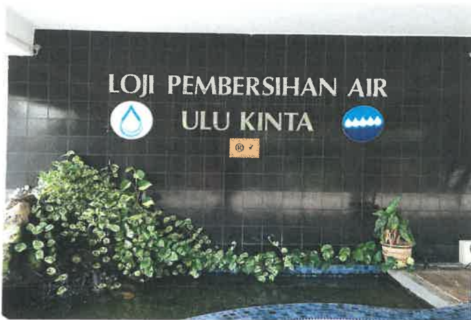
Figure 4.1 : Ulu Kinta Wastewater Treatment Plant
