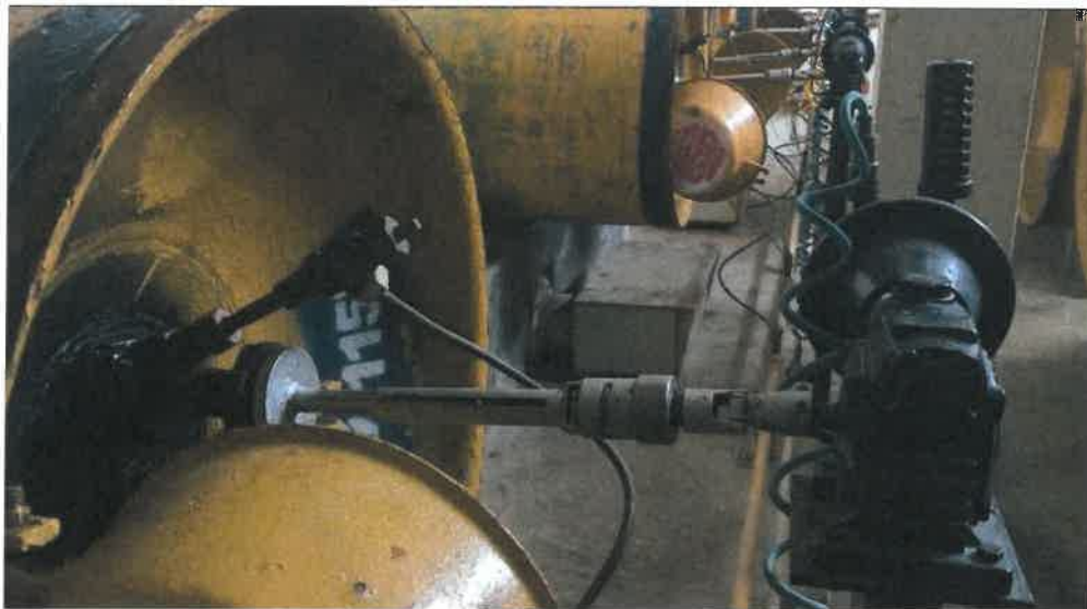
Figure 4.8 : Installation of chlorine drum
