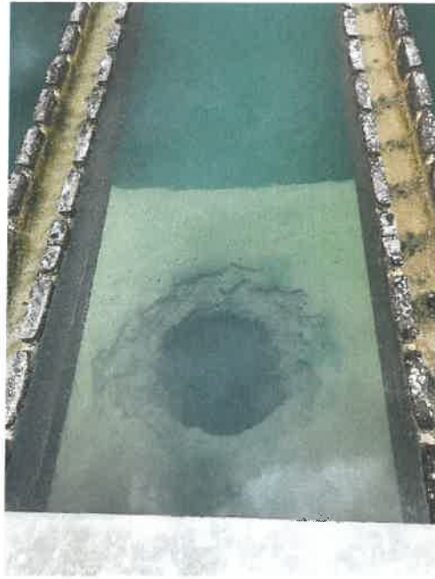
Figure 4.7 : The sludge blanket that has been produced
