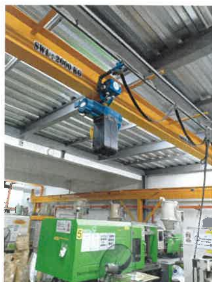
Crane used to lift mold
