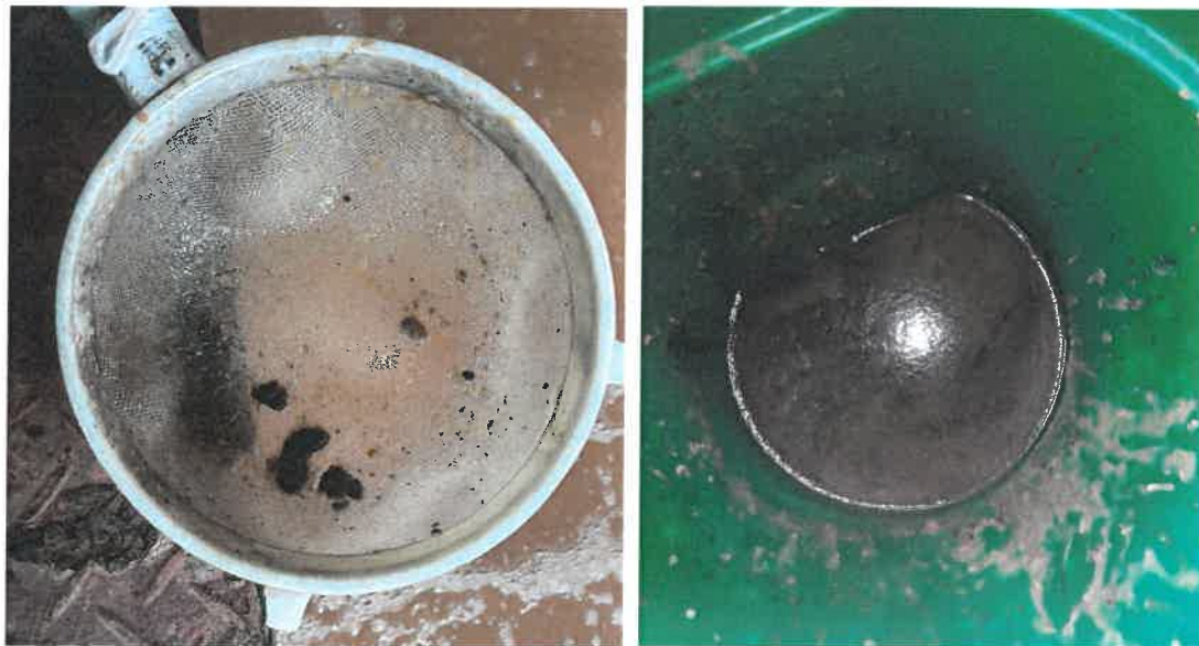
Figure 17: The clack sludge found in aeration tank 2
