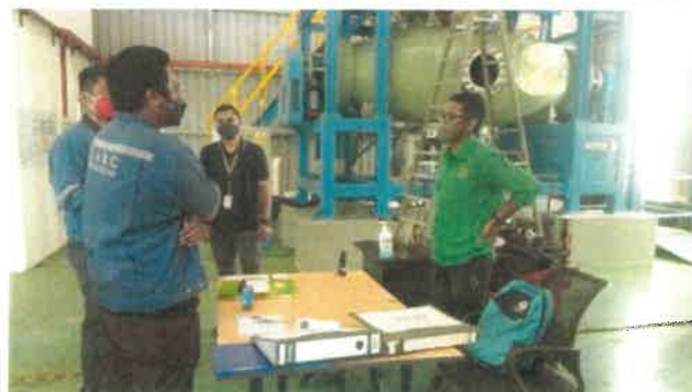
Appendice 1 : Boiler and MRM inspection with OSHA officer.
