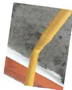
Figure 4: Repainting Pipe with Yellow
