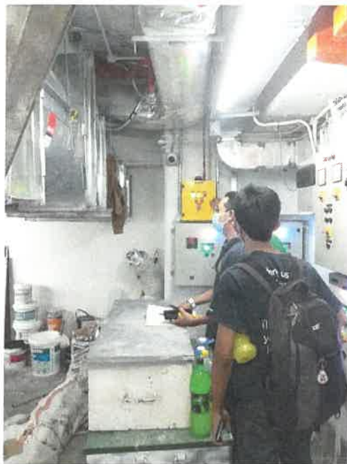
Figure 18: Site visit to Nanyang Coffee @ Midvalley
