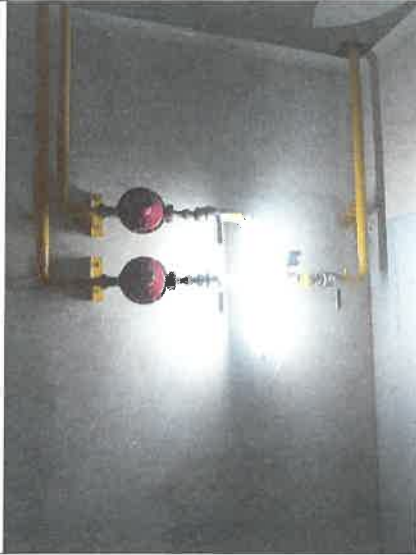
Main Pipe's Installation
